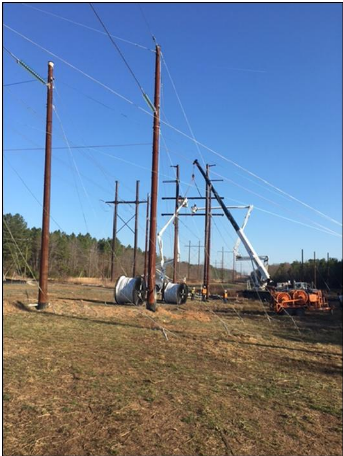
Removal of H-Frame Switch Structure at the North Doswell DP Tap
