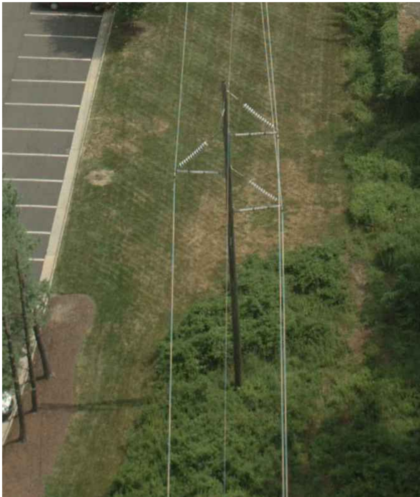
LOOKING NORTHEAST — EXISTING TRANSMISSION STRUCTURE #2010/12 — 61'± HIGH SINGLE CIRCUIT WOOD POLE
