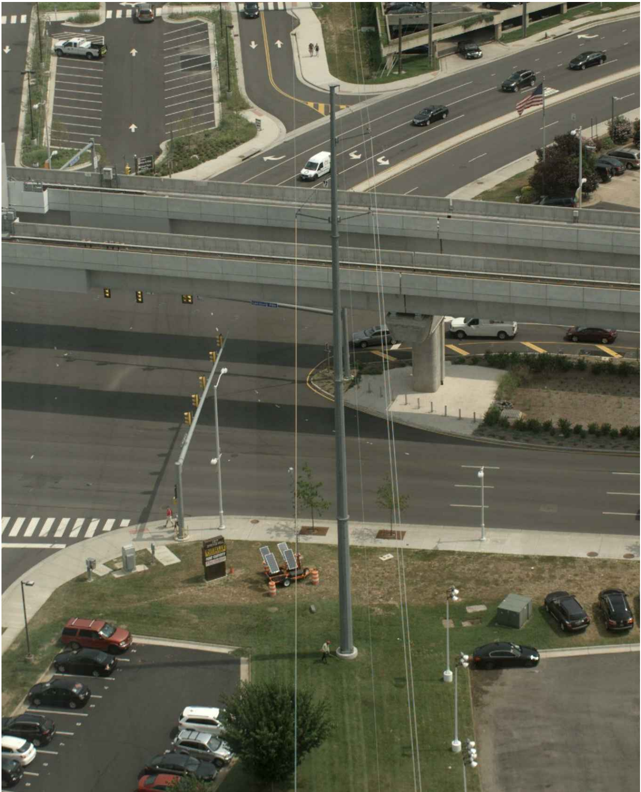
LOOKING NORTHEAST — EXISTING TRANSMISSION STRUCTURE #2010/6 — 140'± HIGH SINGLE CIRCUIT STEEL POLE
