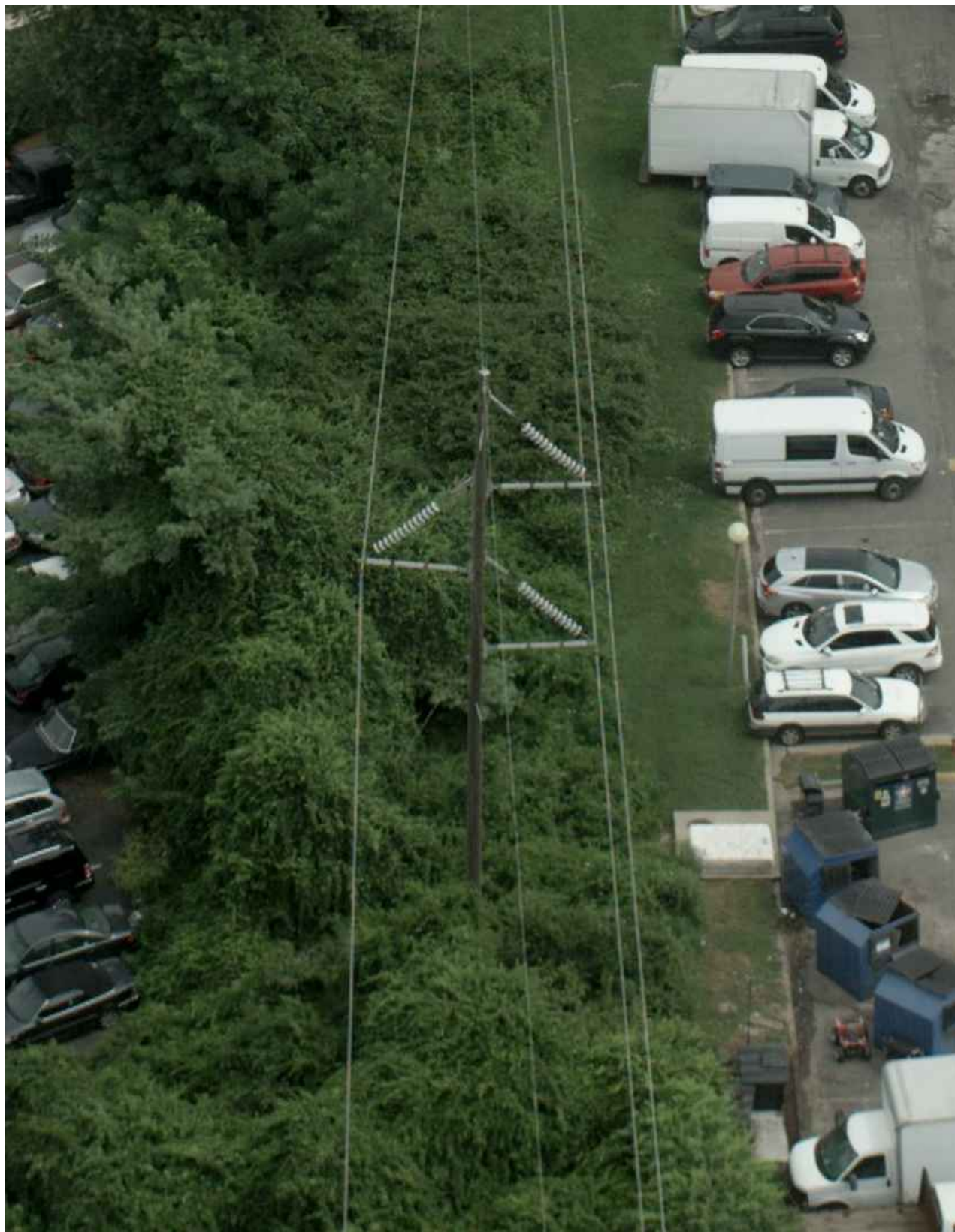
LOOKING NORTHWEST – EXISTING TRANSMISSION STRUCTURE #2010/3 – 65.5'± HIGH SINGLE CIRCUIT WOOD POLE
