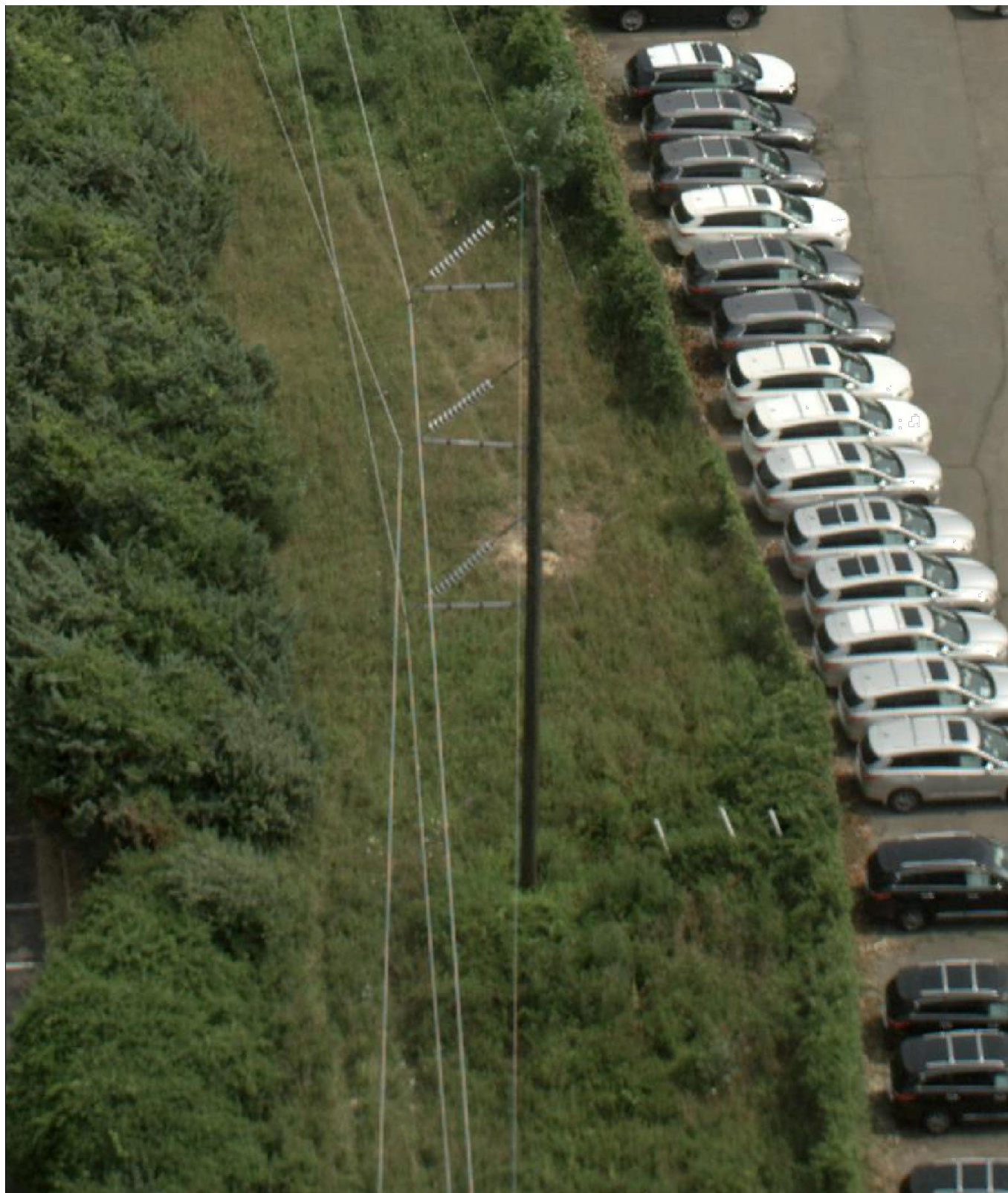
LOOKING NORTHEAST – EXISTING TRANSMISSION STRUCTURE #2010/11 – 65.5'± HIGH SINGLE CIRCUIT WOOD POLE
