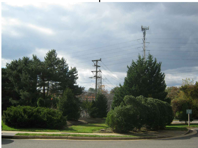
HOLLY MANOR DRIVE/ SHREVE RD INTERSECTION
