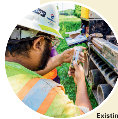
Dominion Energy image. Not project specific.
