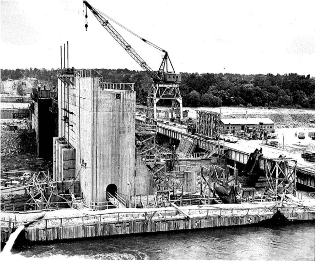
*To get more energy from the river, a tailrace was constructed. Construction involved blasting and removing solid bedrock, 40' deep by 60' wide, for about 1.2 miles. This gave the dam a higher "head" which gave the turbine-generators about 20 percent more generating capacity.*
