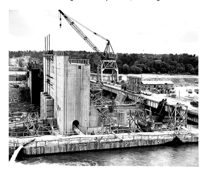
To get more energy from the river, a tailrace was constructed. Construction involved blasting and removing solid bedrock, 40' deep by 60' wide, for about 1.2 miles. This gave the dam a higher "head" which gave the turbinegenerators about 20 percent more generating capacity.
