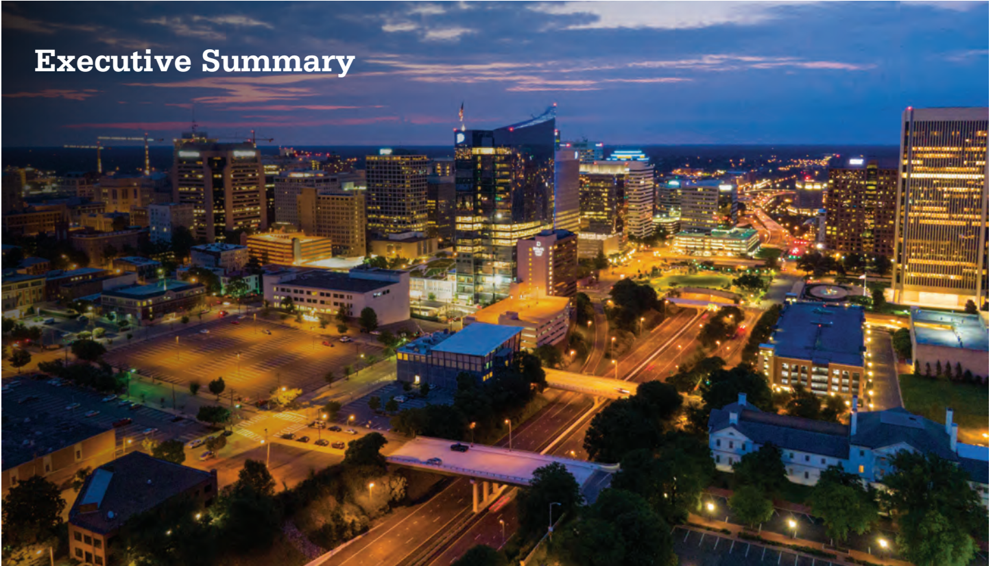
Dominion Energy Corporate Office; Thomas F. Farrell building; Richmond, VA
