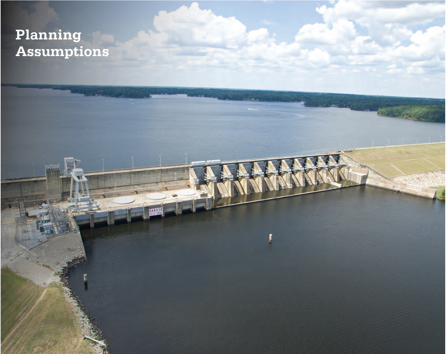
Gaston Hydro Station; Theima, NC
