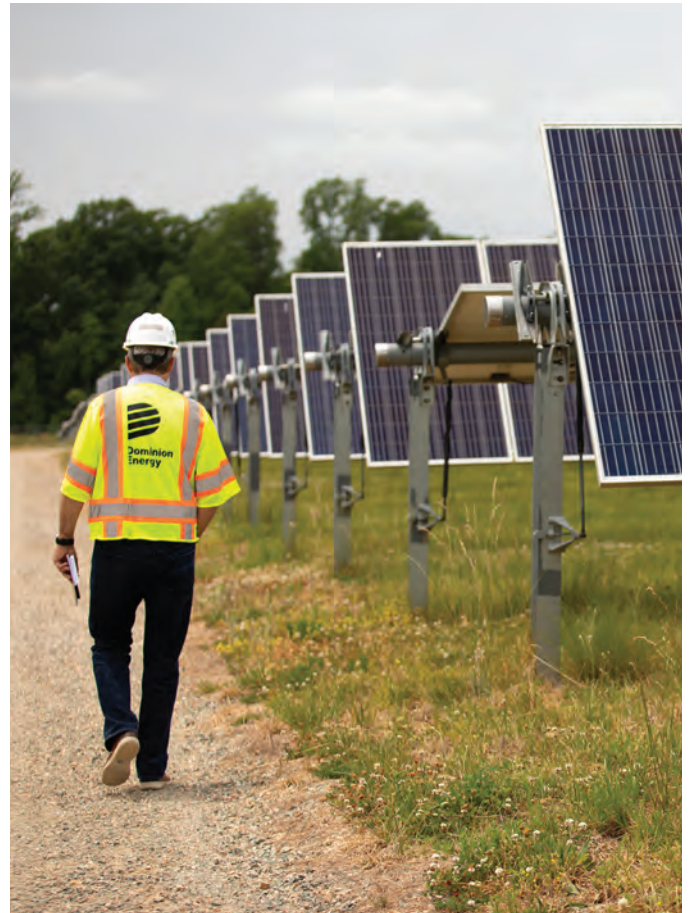
Scott Solar Facility; Powhatan County, VA
