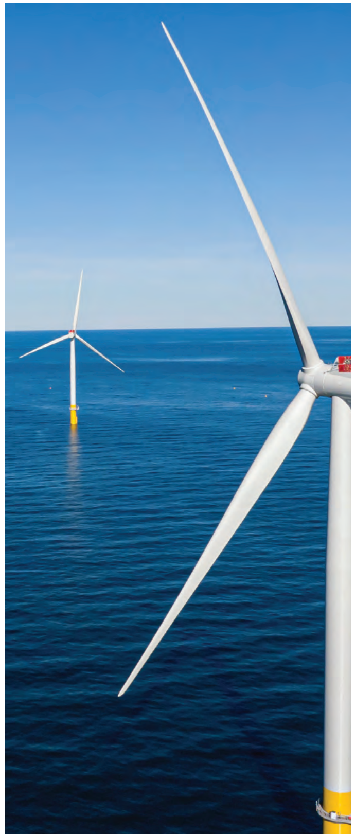
Dominion Energy's Coastal Virginia Offshore Wind Project
