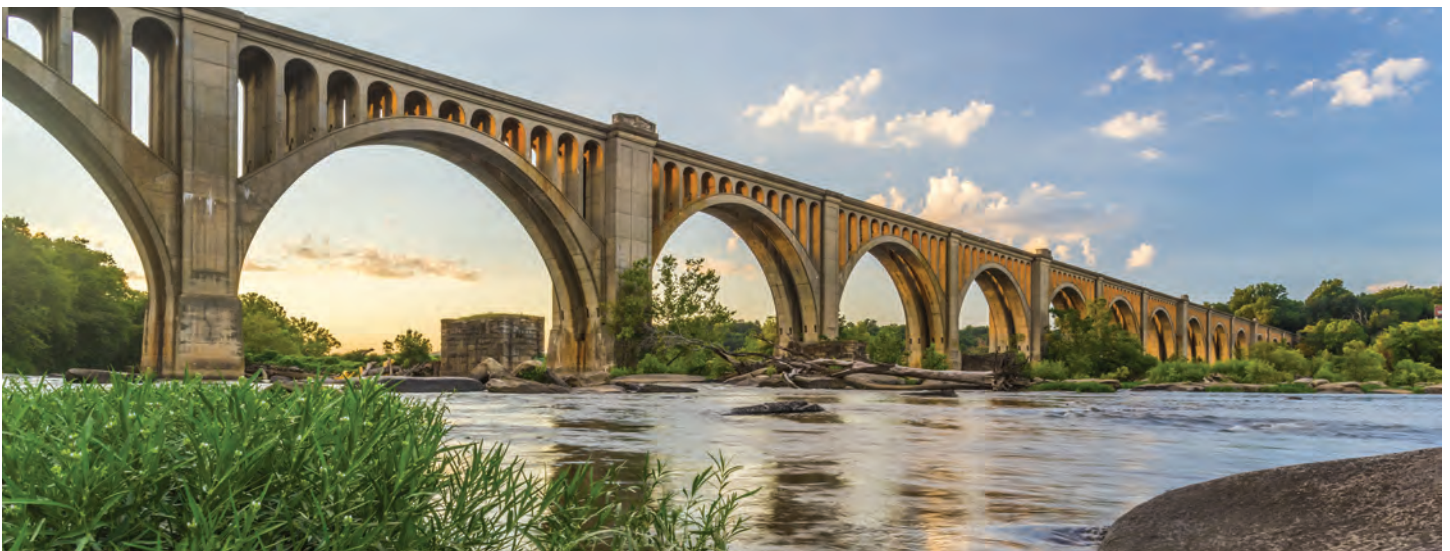
This concrete arch railroad bridge spanning the James River; Richmond, VA
