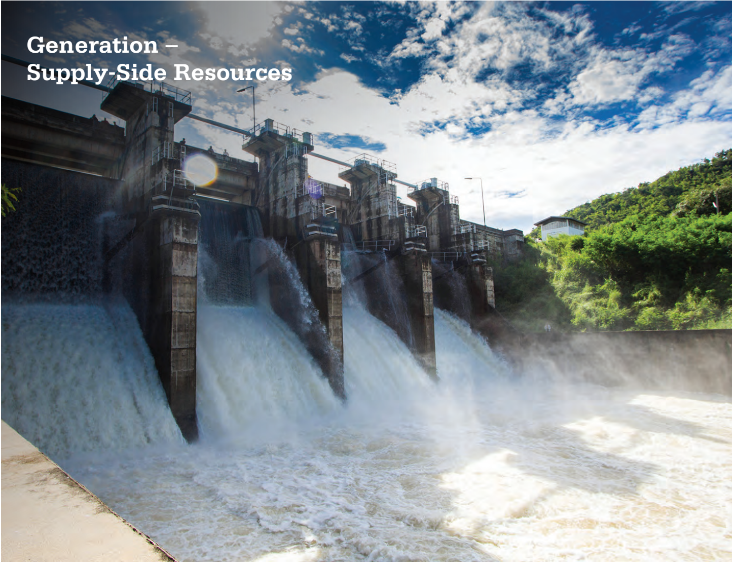
North Anna Hydro Power Plant
