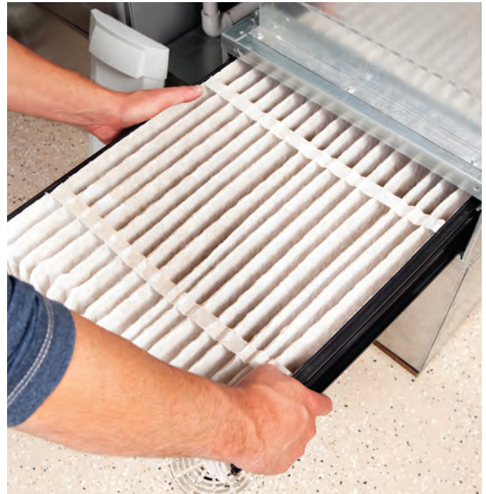
Air filter replacement in an HVAC unit
