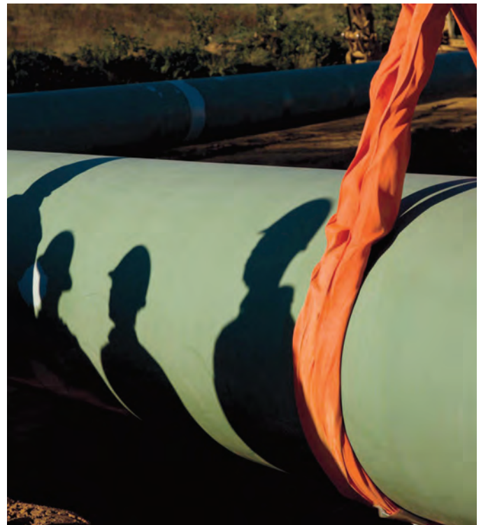
Natural Gas pipeline installation
