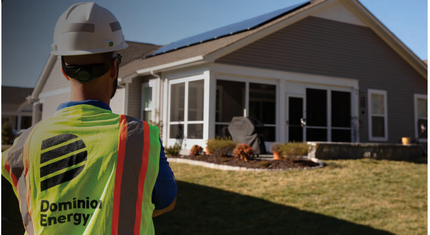
BrightSuite solar install
