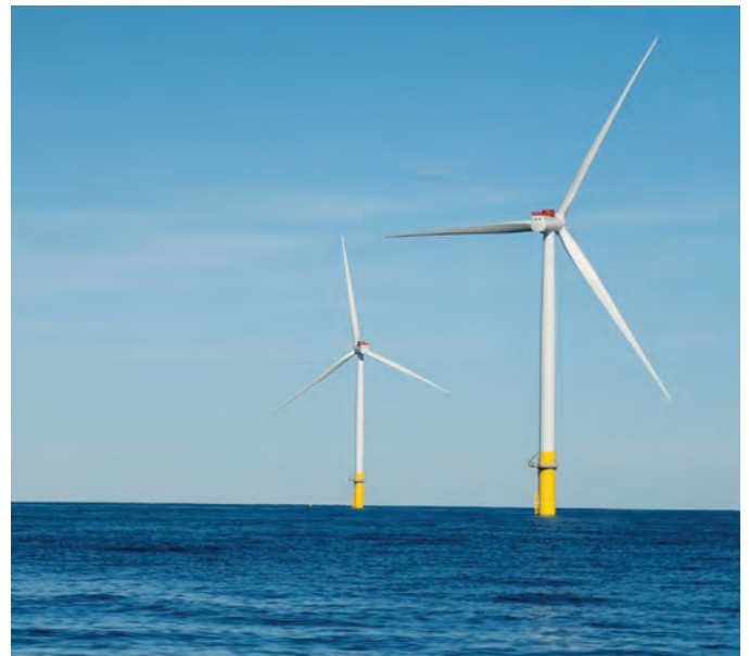
Dominion Energy's Coastal Virginia Offshore Wind Project
