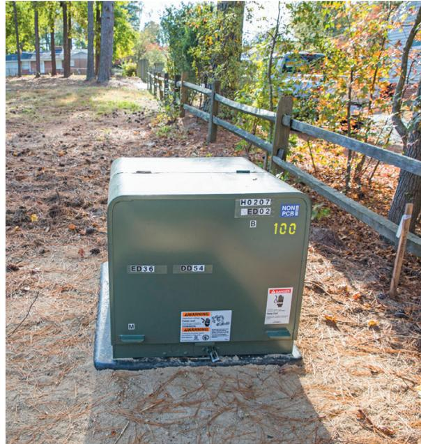
Single-phase transformers supply power for residential lighting, receptacles, air-conditioning and heating. Average transformer size: 40" wide x 36" deep x 34" high.
