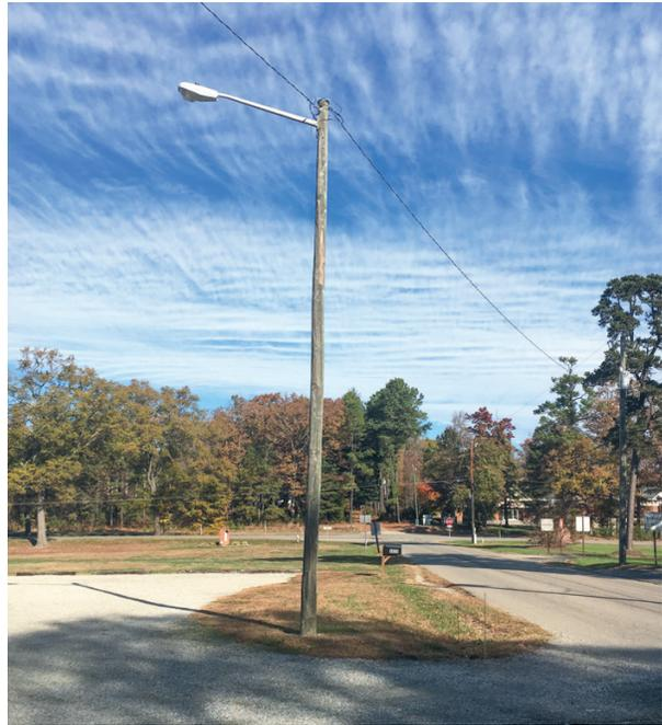
An Enclosed Drop Lens fixture on a wood pole
