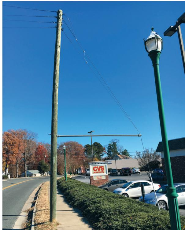
A down guy maybe needed to help support the load on a pole. Down guys typically anchor in the ground a minimum of 15 feet from the pole.
