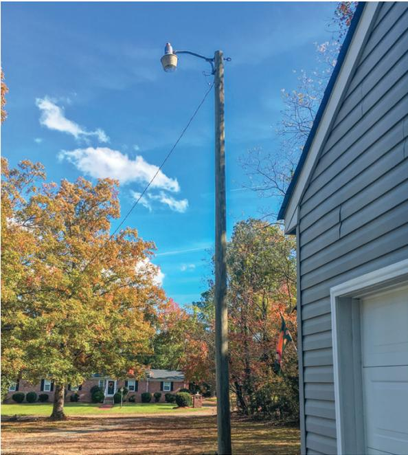
An Open Vertical fixture on a wood pole
