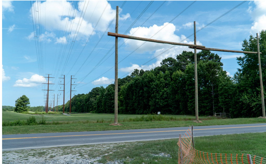
Representative photo of a typical wooden guard structure.
