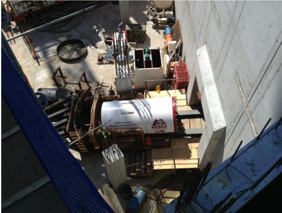
Figure 9 – Microtunneling from deep building excavation.
