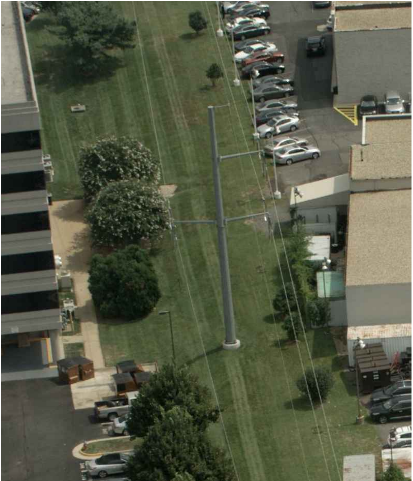
LOOKING NORTHEAST – EXISTING TRANSMISSION STRUCTURE #2010/7 – 70'± HIGH SINGLE CIRCUIT STEEL POLE
