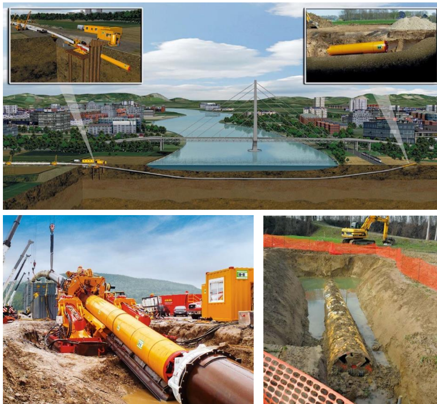
Figure 11 Direct pipe (images from Herrenknecht)
