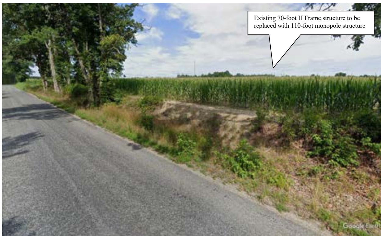
Figure 5-8: View 6- View from Woodford Road 0.15 mile west of Braynefield property towards the project alignment, facing northwest. (One existing structure to be replaced is visible across field)
