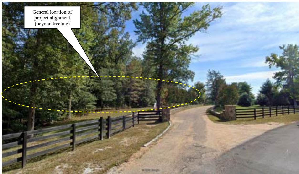
Figure 5-12: Photo location 1- View of Edge Hill setting from Edge Hill Academy Road, facing south.
