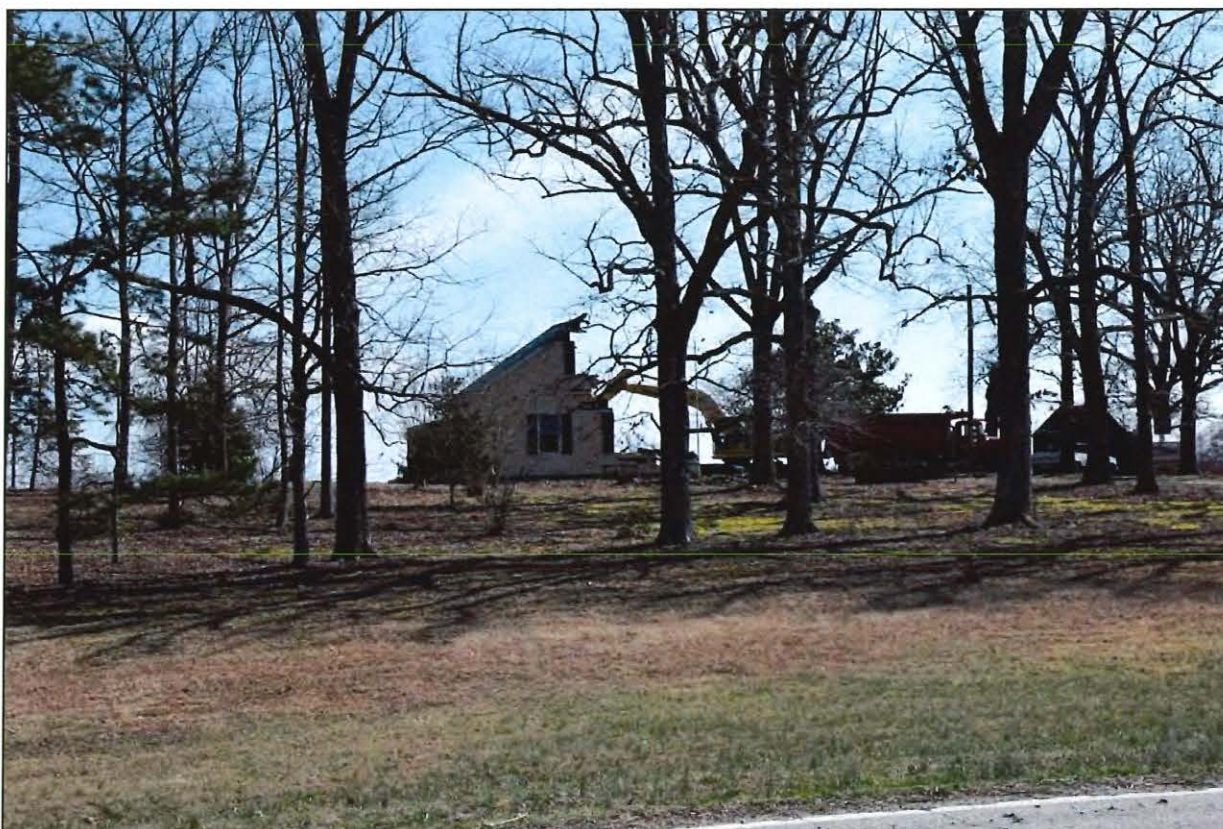
Figure 4. 058-0131, Red Fox Farm, dwelling, view east-southeast along Route 688.
