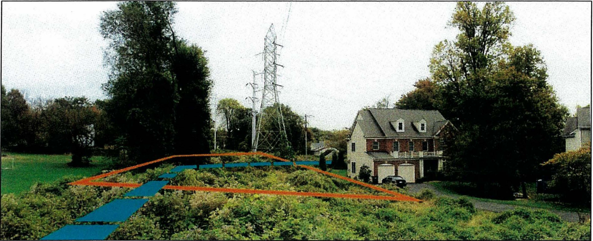
Figure 3.6.1-4. Photograph illustrating the route of Underground Alternative 04 showing the temporary HDD workspace east of I-66 and north of Idylwood substation, with no tree removal within 053-0276 (Photo view 11).
