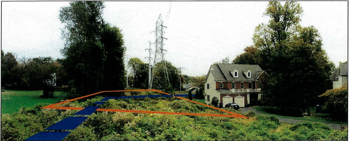
Figure 3.8.1-4. Photograph illustrating the route of Underground Alternative 06 showing temporary HDD workspace east of I-66 and north of Idylwood substation, with no tree removal within 053-0276 (Photo view 15).
