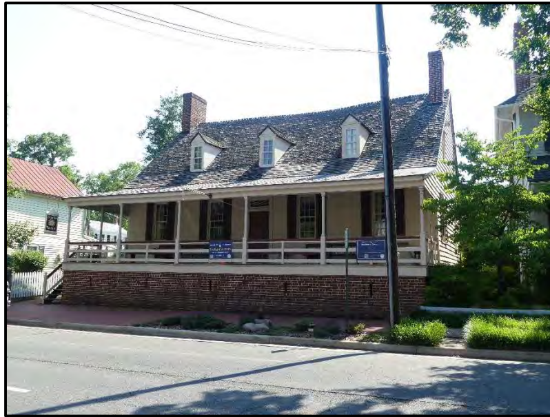
Figure 55 View of Eagle Tavern / Rising Sun Tavern (DHR # 111-0088), Looking Southwest.
