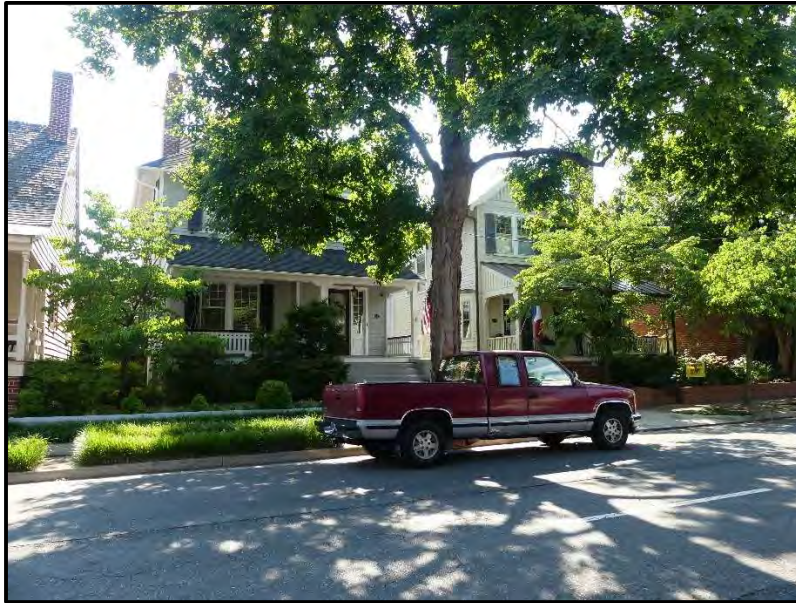
Figure 56 View of Eagle Tavern / Rising Sun Tavern (DHR # 111-0088), Towards Transmission Line Looking West (Photo Location 7)
