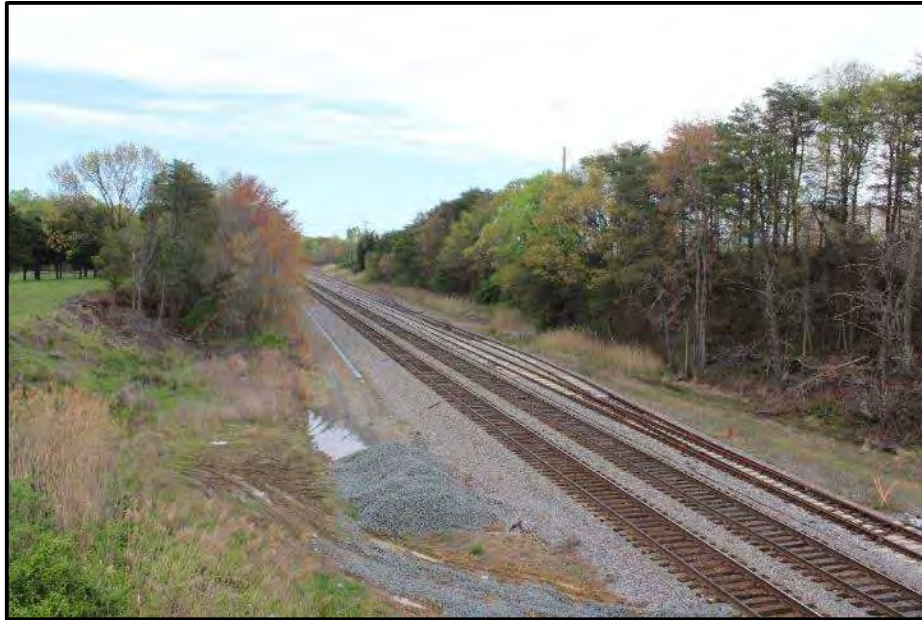
Figure 17 View of Richmond, Fredericksburg & Potomac Railroad (DHR #076-0301), Richmond, Fredericksburg & Potomac Railroad Historic District (DHR #500-0001), and the Cockpit Point Battlefield (DHR #076-5842; Photo Location 2) Looking North/Northeast.
