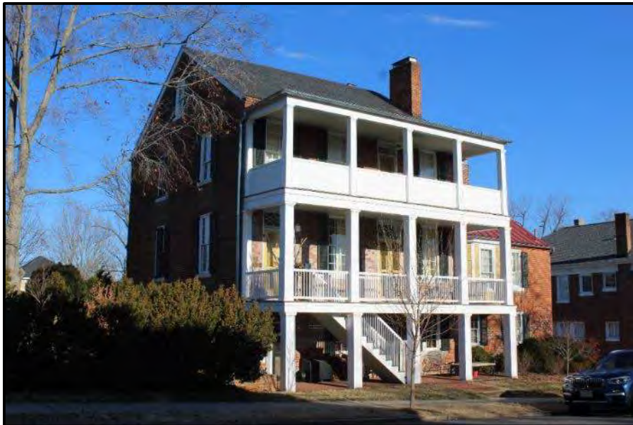
Figure 31 View of John Lewis House/Rowe House/War Hospital (DHR #111-0107), Looking North.
