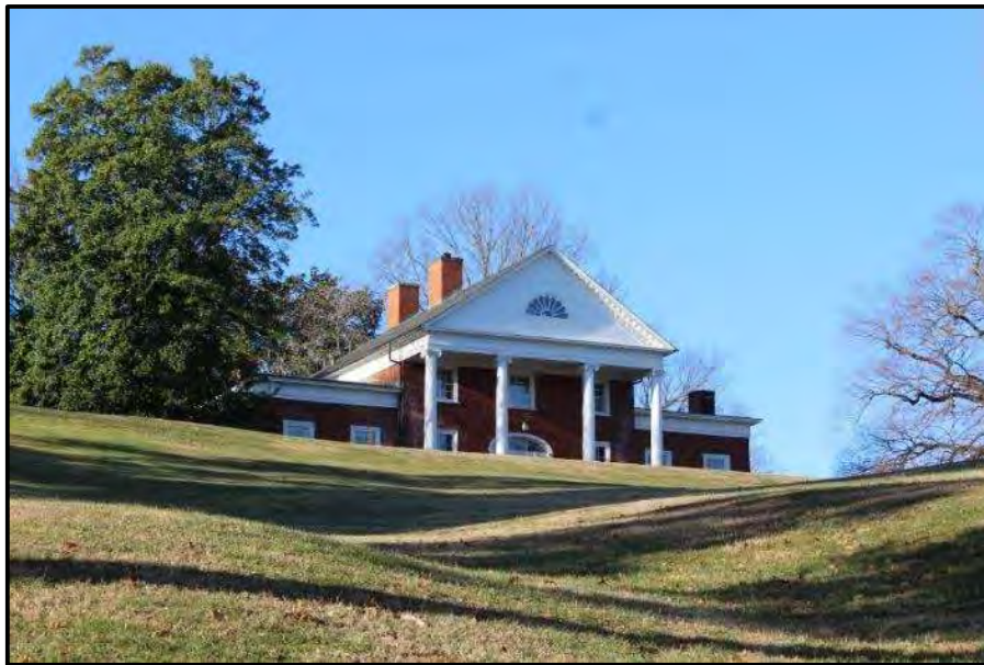
Figure 25 View of Brompton (DHR #111-0008), Looking West.
