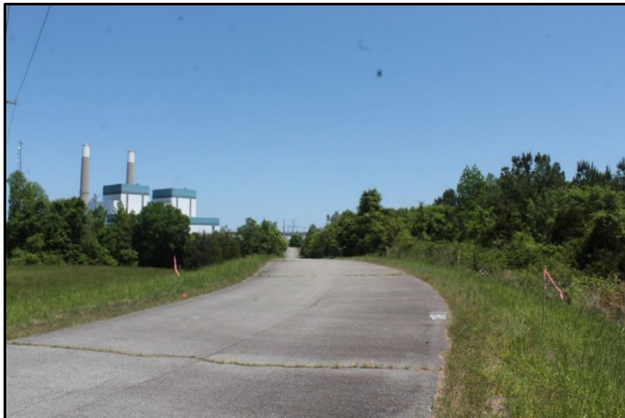
Figure 20 View from Staunton River Bridge Battlefield (DHR #019-5190) Looking Northeast (Photo Location 7). Clover Substation is Visible. Structure in Center of Photograph is not Part of the Current Project.
