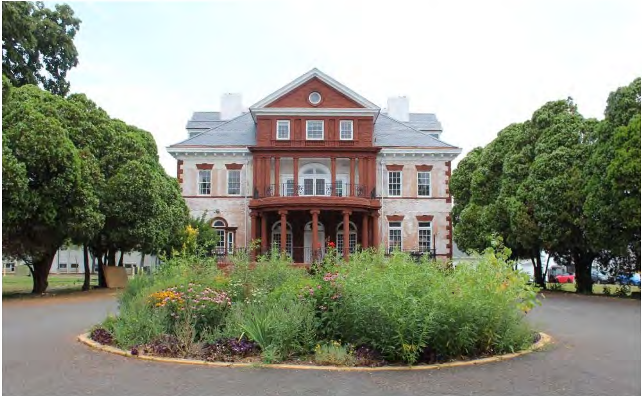
Figure 5-82: Photo location 1- Representative view of Annaburg front facade, facing northeast.
