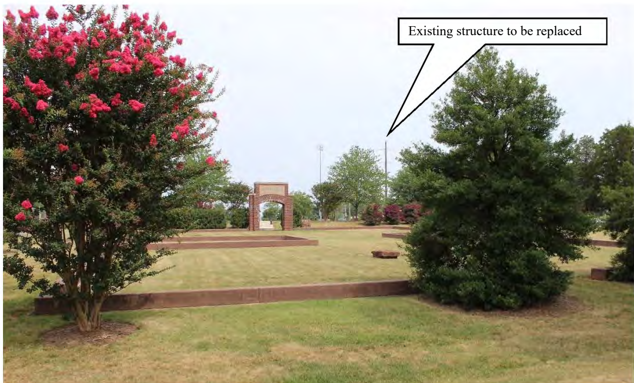
Figure 5-74: Photo location 6- View from south edge of site (One project structure visible), facing north.
