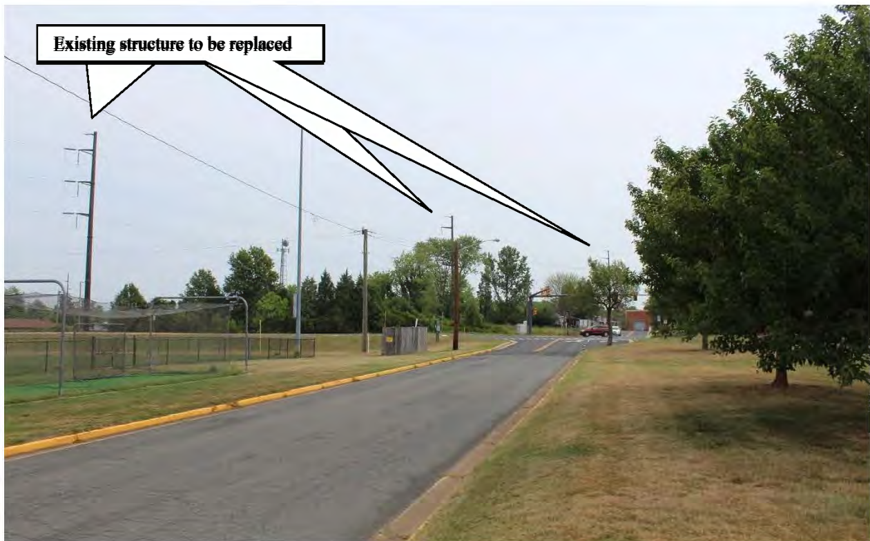
Figure 5-183: Photo location 4- View from Jennie Dean Memorial Site (Multiple project structures visible), facing northeast.
