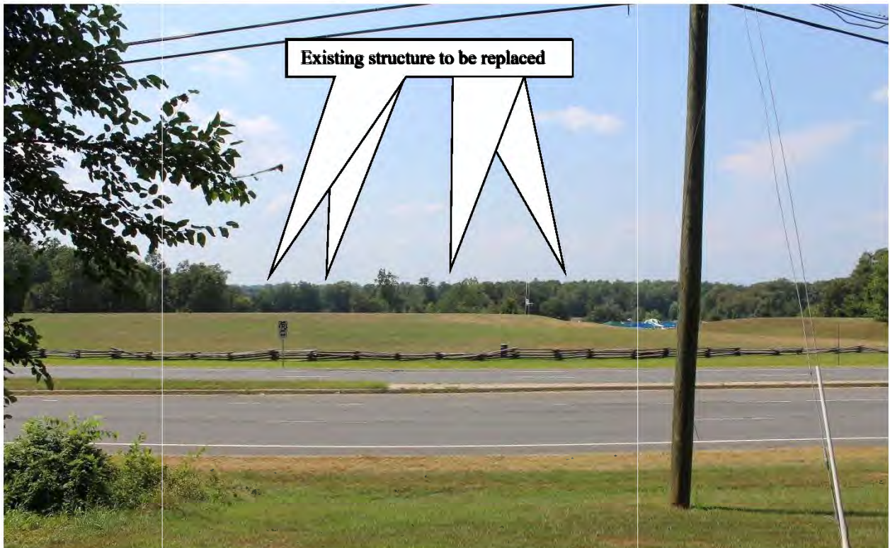
Figure 5-14: Photo location 2- View from Signal Hill (Multiple project structures visible), facing northwest.
