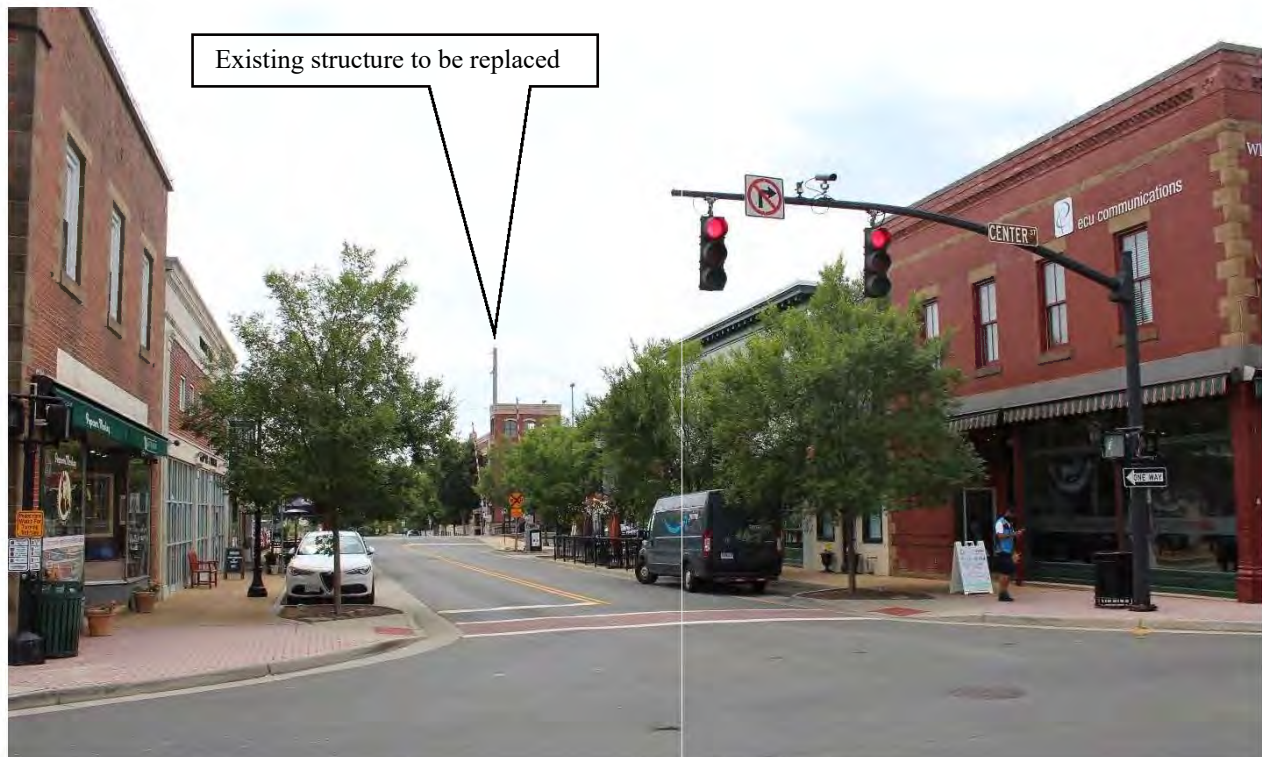
Figure 5-110: Photo location 6- View from Center Street at Main Street (Project structure visible), facing south.
