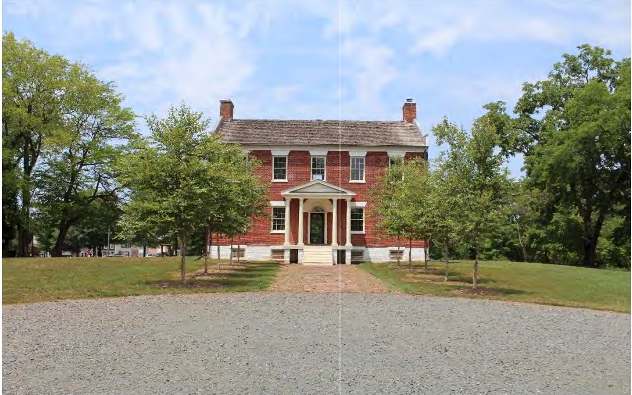
Figure 5-60: Photo location 1- Representative view of Liberia front facade, facing northwest.
