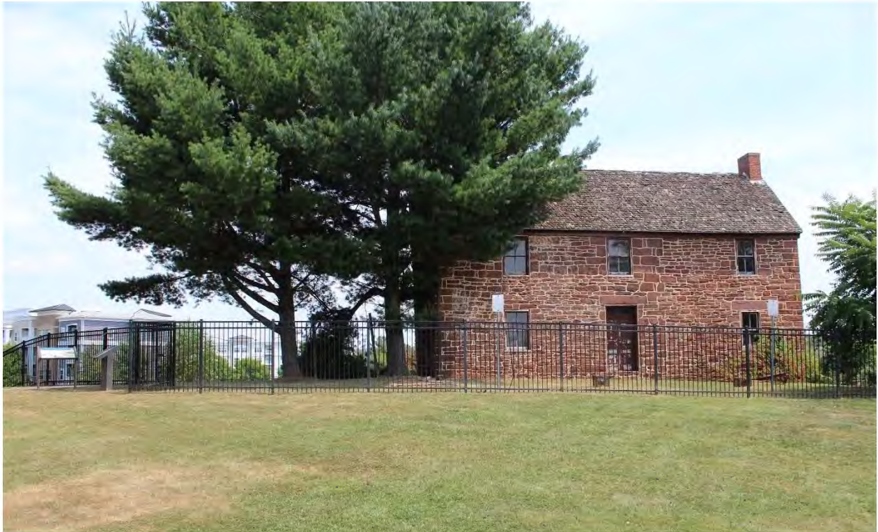
Figure 5-38: Photo location 1- Representative view of Conner House front facade, facing east.
