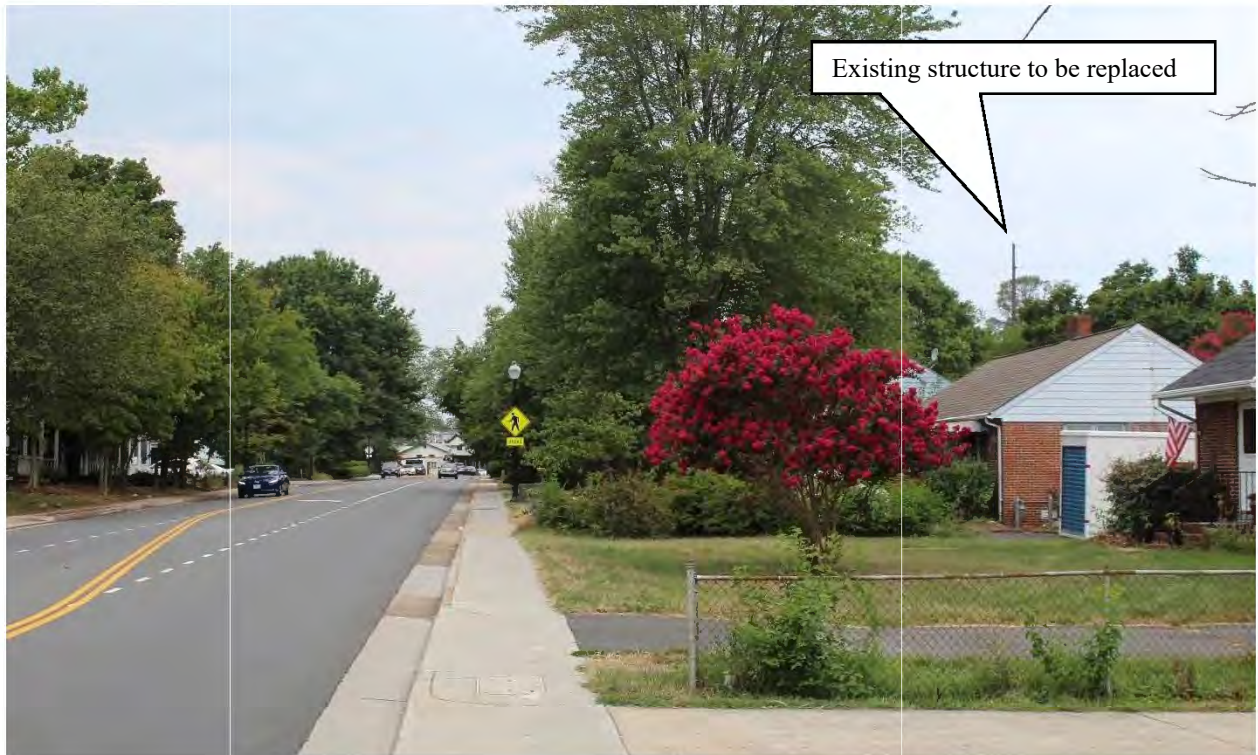
Figure 5-115: Photo location 11- View from Fairview Avenue south of railroad (Project structure visible), facing north.
