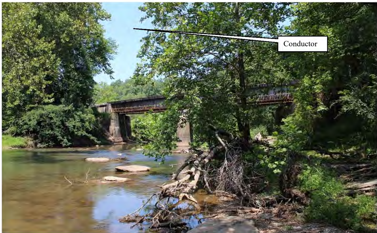
Figure 5-195: Photo location 16 - Representative view of existing bridge from hiking trail along Bull Run Creek (Conductor visible above bridge but no project structures visible), facing north.
