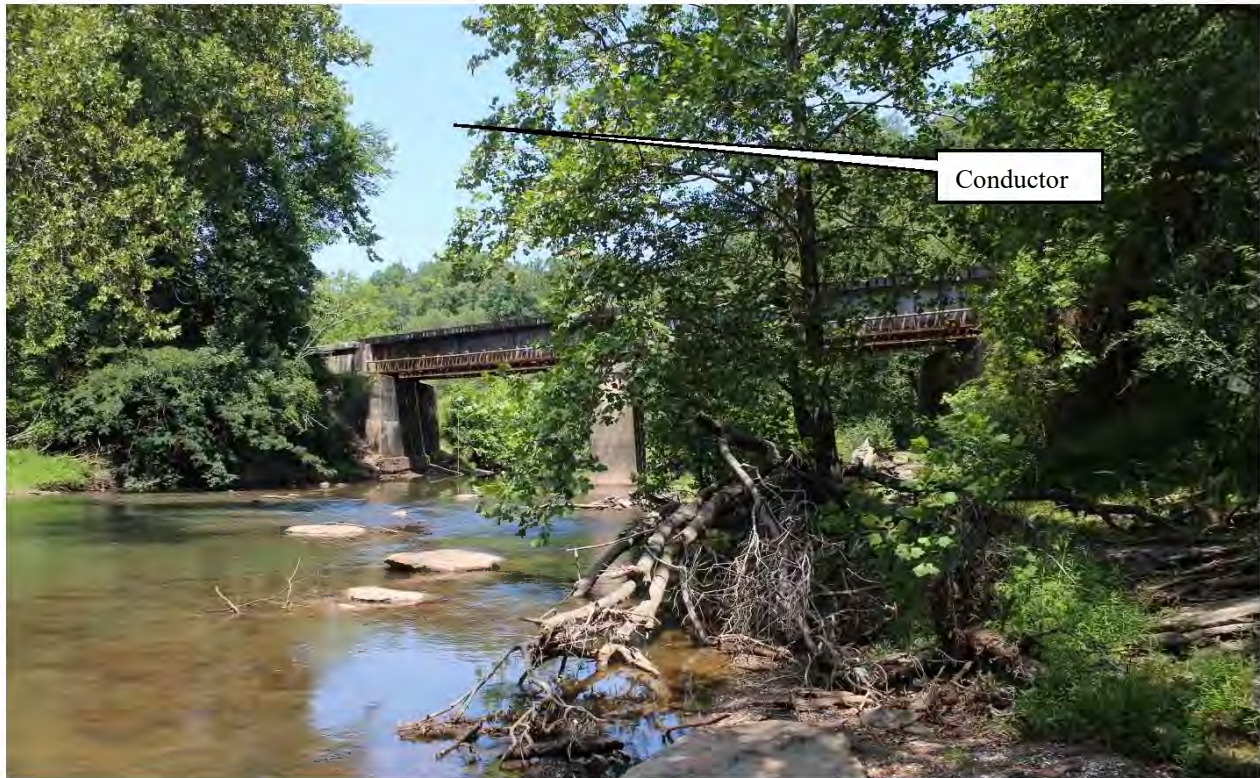
Figure 5-20: Photo location 1- Representative view of existing bridge from hiking trail along Bull Run Creek (conductor visible above bridge but no project structures visible), facing north.
