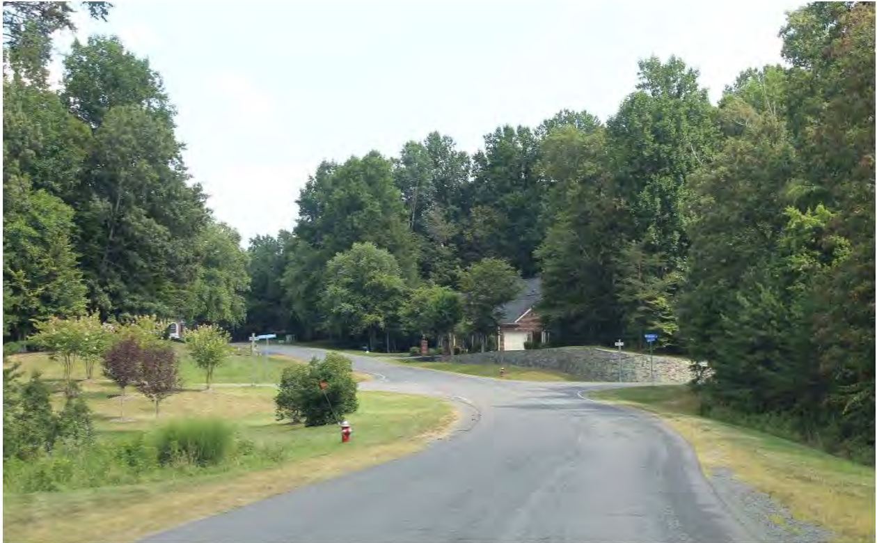
Figure 5-259: Photo location 1- Representative view of Union Mills Historic District along Balmoral Greens Road, facing east.
