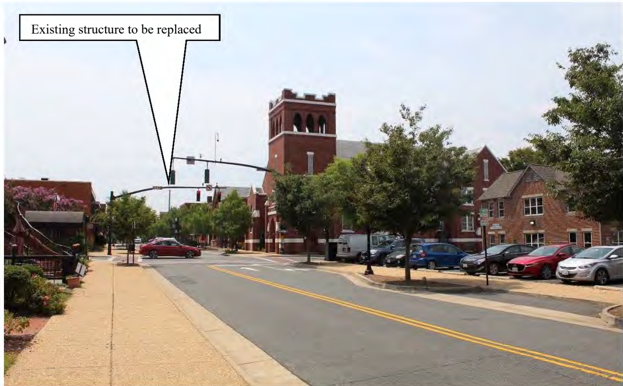
Figure 5-119: Photo location 15 - View from Main Street at Church Street (Project structure visible), facing south.
