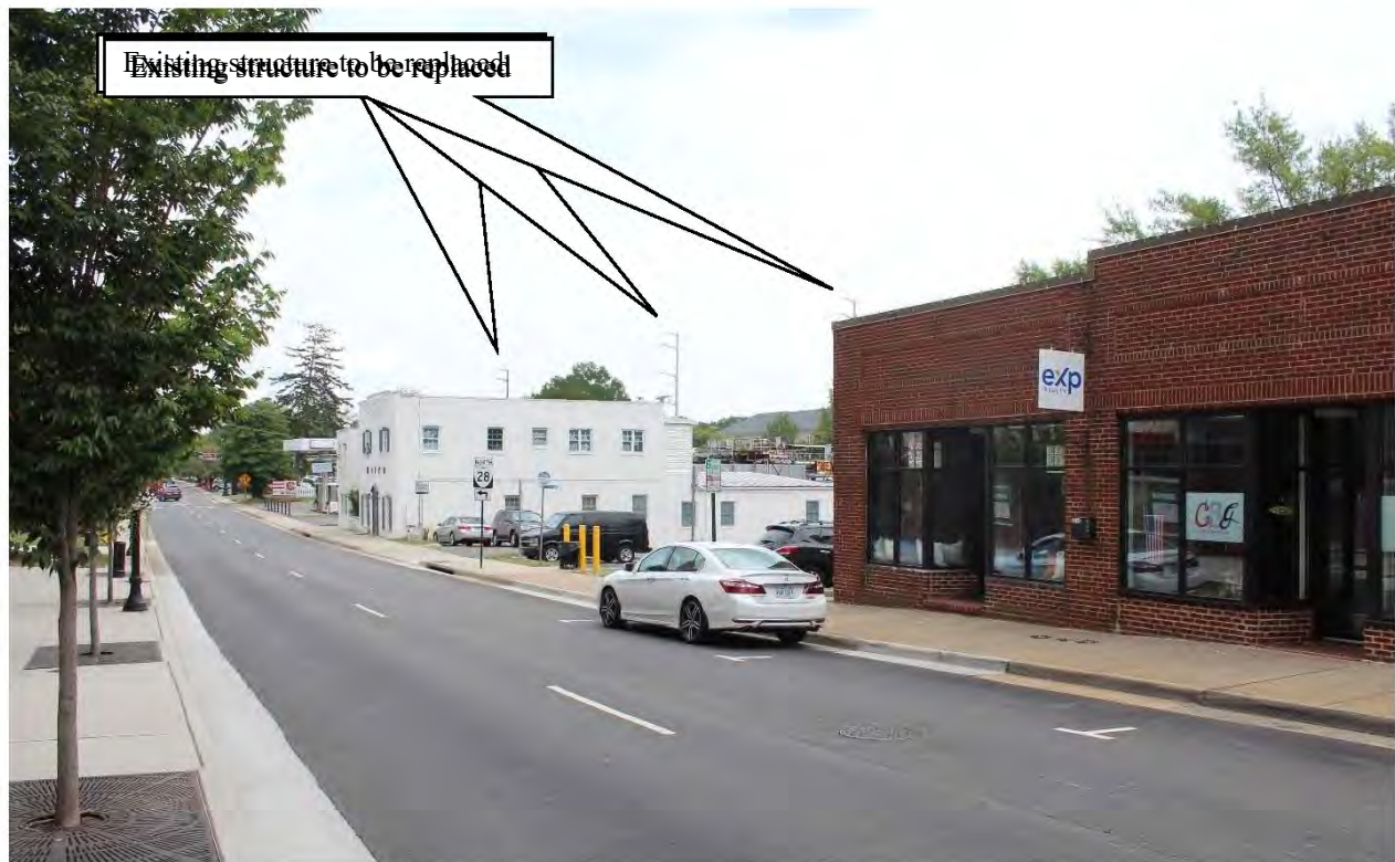
Figure 5-112: Photo location 8- View from Center Street east of East Street (Multiple project structures visible), facing southeast.
