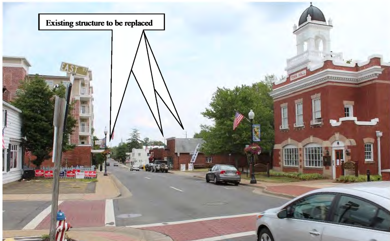
Figure 5-111: Photo location 7- View from Center Street at East Street (Multiple project structures visible), facing east.
