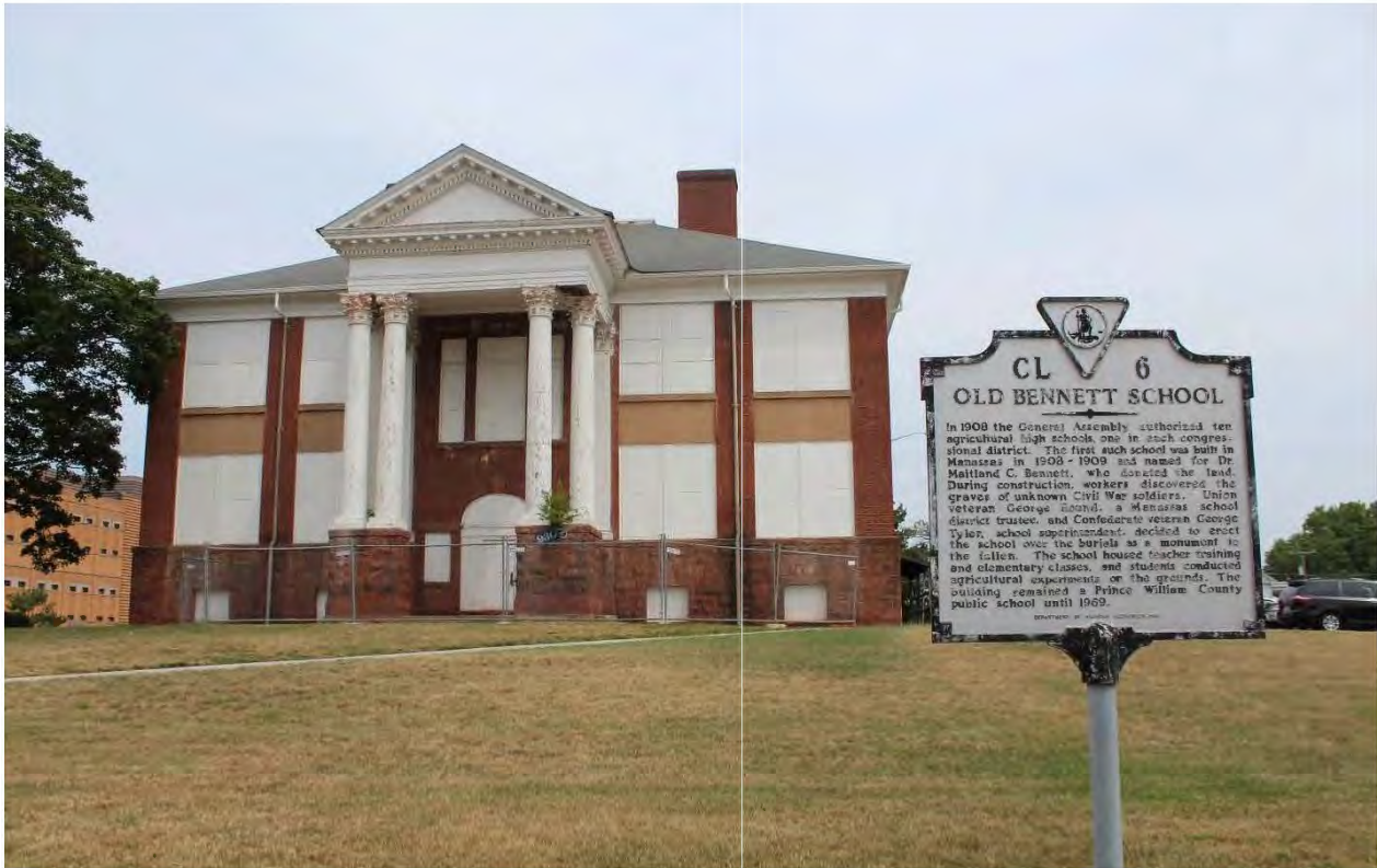
Figure 5-273: Photo location 1- Representative view of Bennett School front facade, facing north.
