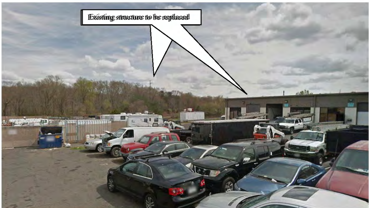
Figure 5-242: Photo location 4- View from Industry Drive (Several project structures visible), facing southeast.
