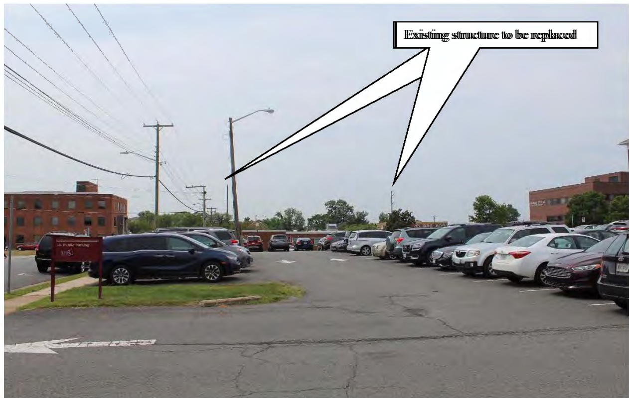
Figure 5-276: Photo location 4- View from parking lot to rear of Bennett School (Two existing project structures visible), facing south.
