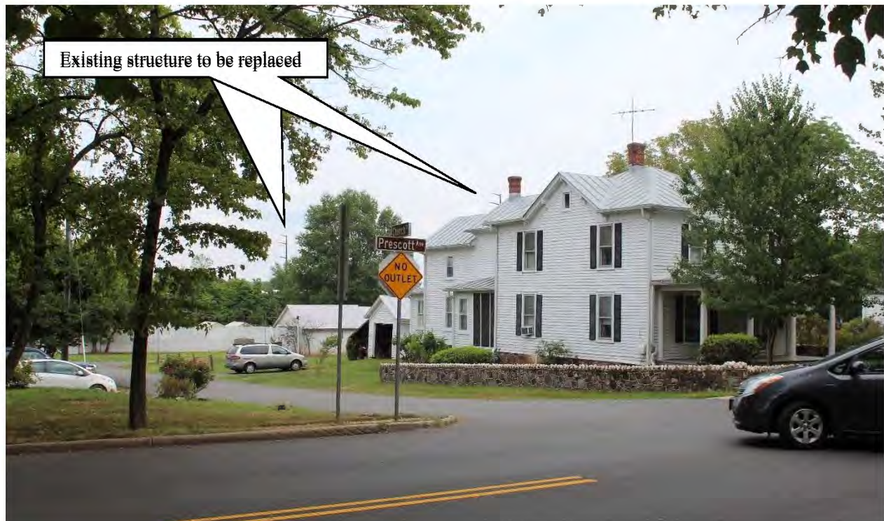
Figure 5-117: Photo location 13- View from Prescott Avenue at Church Street (Multiple project structures visible), facing south.
