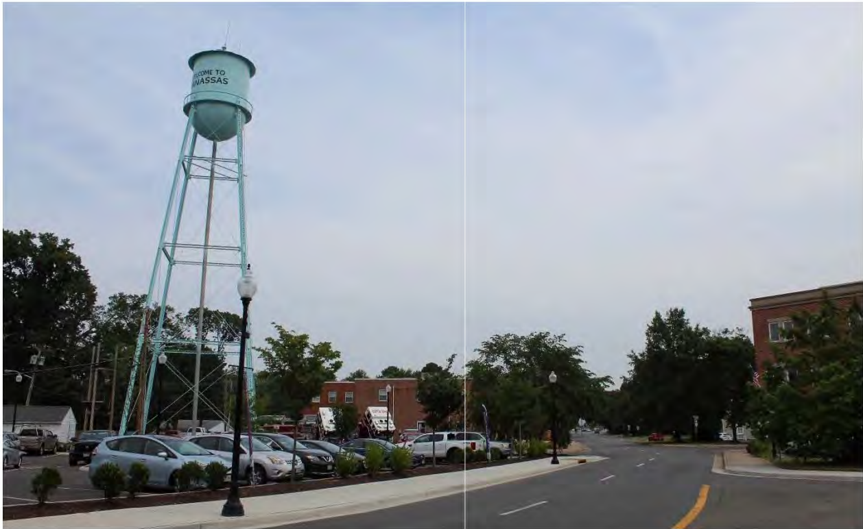
Figure 5-97: Photo location 1- Representative view of water tower and setting, facing northeast.
