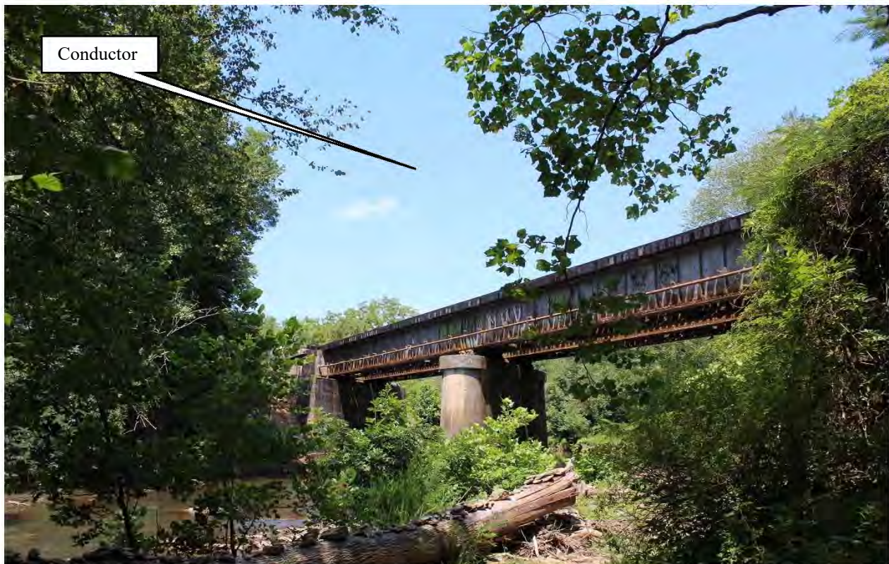
Figure 5-21: Photo location 2- View from trail on south side of bridge (Conductor visible above bridge, but no project structures visible), facing northwest
