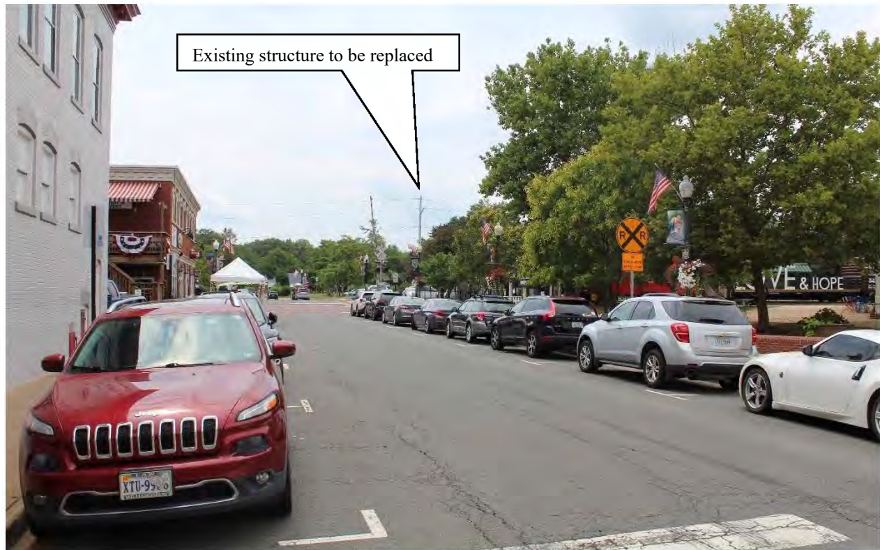
Figure 5-107: Photo location 3- View from West Street at Center Street (Project structure visible), facing south.
