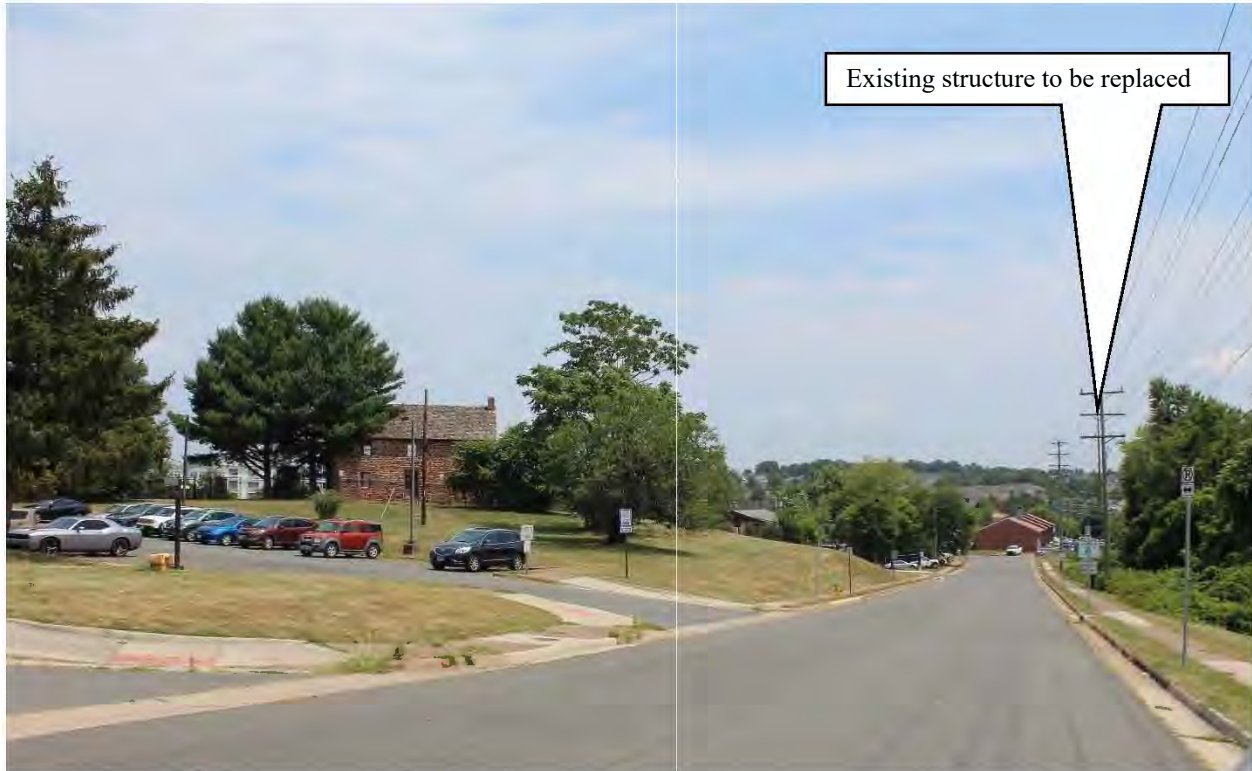
Figure 5-192: Photo location 13- View from Conner House (One project structure visible), facing southeast.
