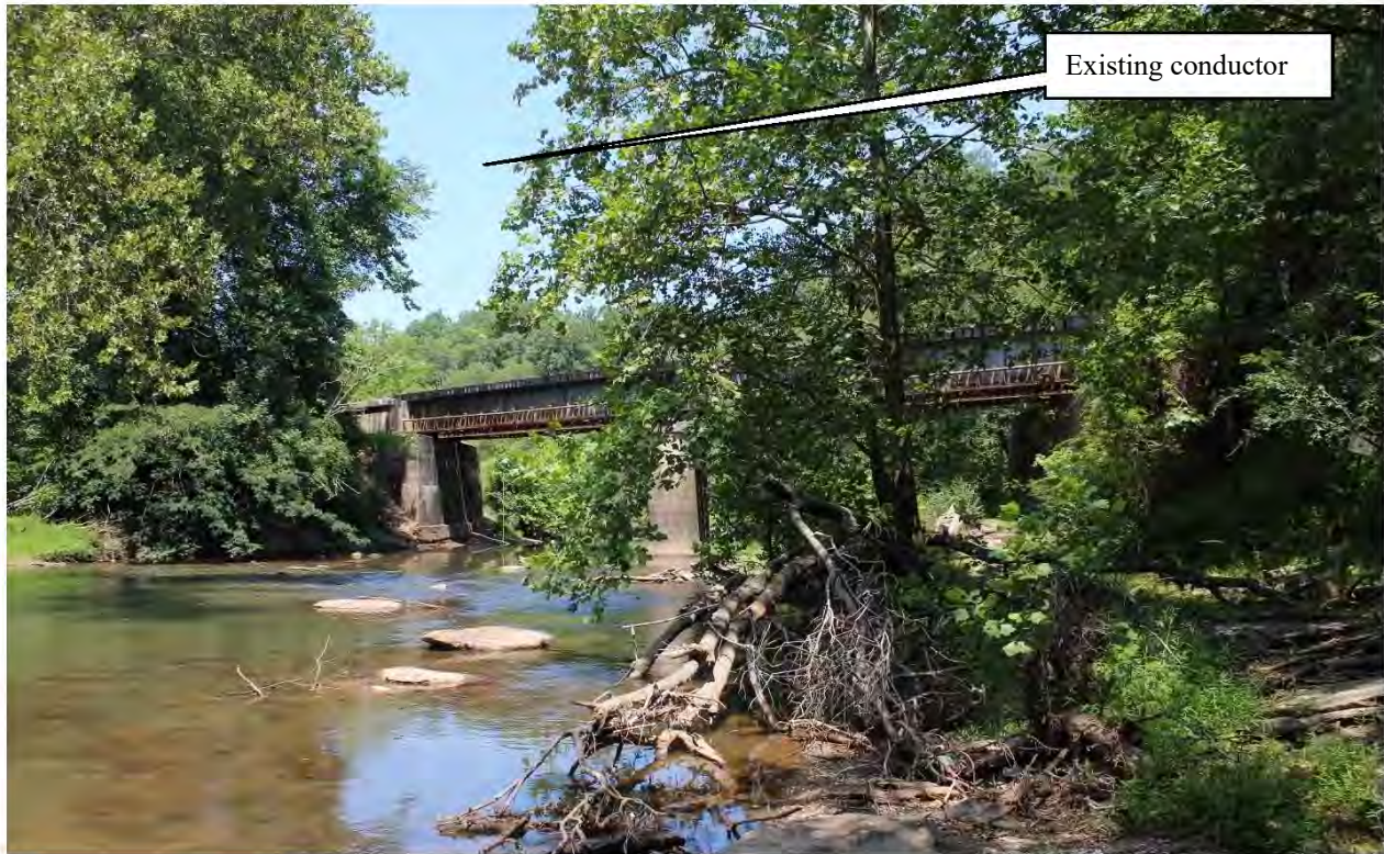
Figure 5-265: Photo location 7- View from O&A Railroad Bridge in Hemlock Regional Park (Existing conductor visible but no project structures visible), facing northwest.
