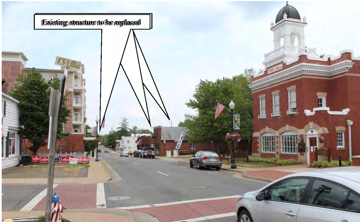
Figure 5-226: Photo location 7- View from Center Street at East Street (Multiple project structures visible), facing east.
