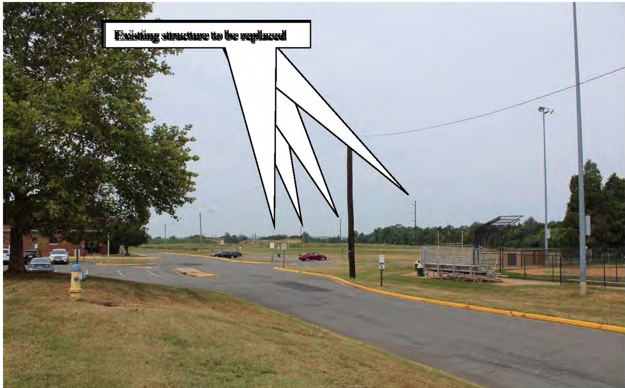
Figure 5-182: Photo location 3- View from Jennie Dean Memorial Site (Multiple project structures visible), facing northwest.
