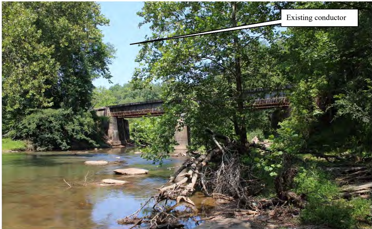
Figure 5-247: Photo location 9- View from O&A Railroad Bridge in Hemlock Regional Park (Existing conductor visible but no project structures visible), facing northwest.
