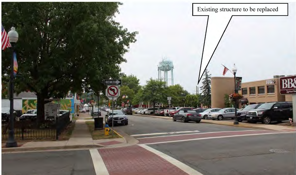
Figure 5-282: Photo location 2- View from vicinity of Pickeral House site (One existing project structure visible), facing south.
