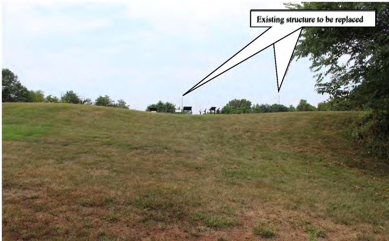
Figure 5-147: Photo location 3- View from trail approaching interpretative area (Multiple project structures visible), facing northwest.
