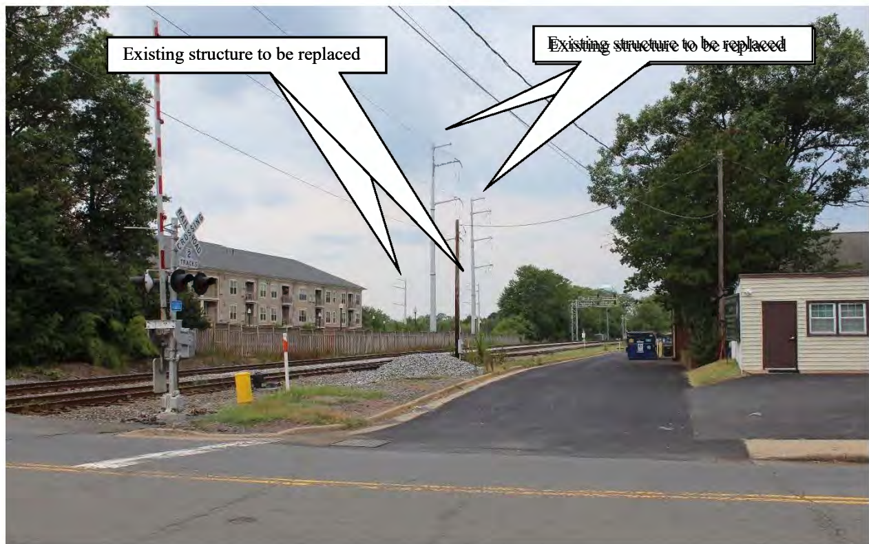
Figure 5-114: Photo location 10- View from Fairview Avenue at railroad crossing (Multiple project structures visible), facing west.
