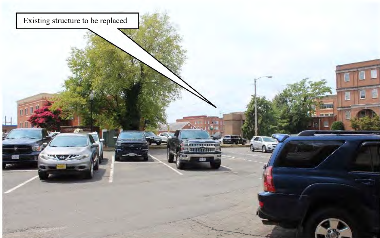
Figure 5-118: Photo location 14- View from Grant Avenue at Mosby Street (Project structure visible), facing south.
