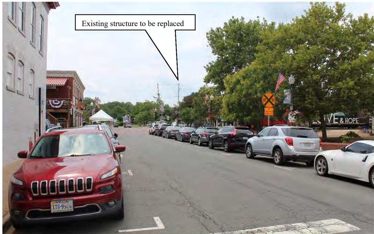
Figure 5-186: Photo location 7- View from West Street at Center Street (Project structure visible), facing south.
