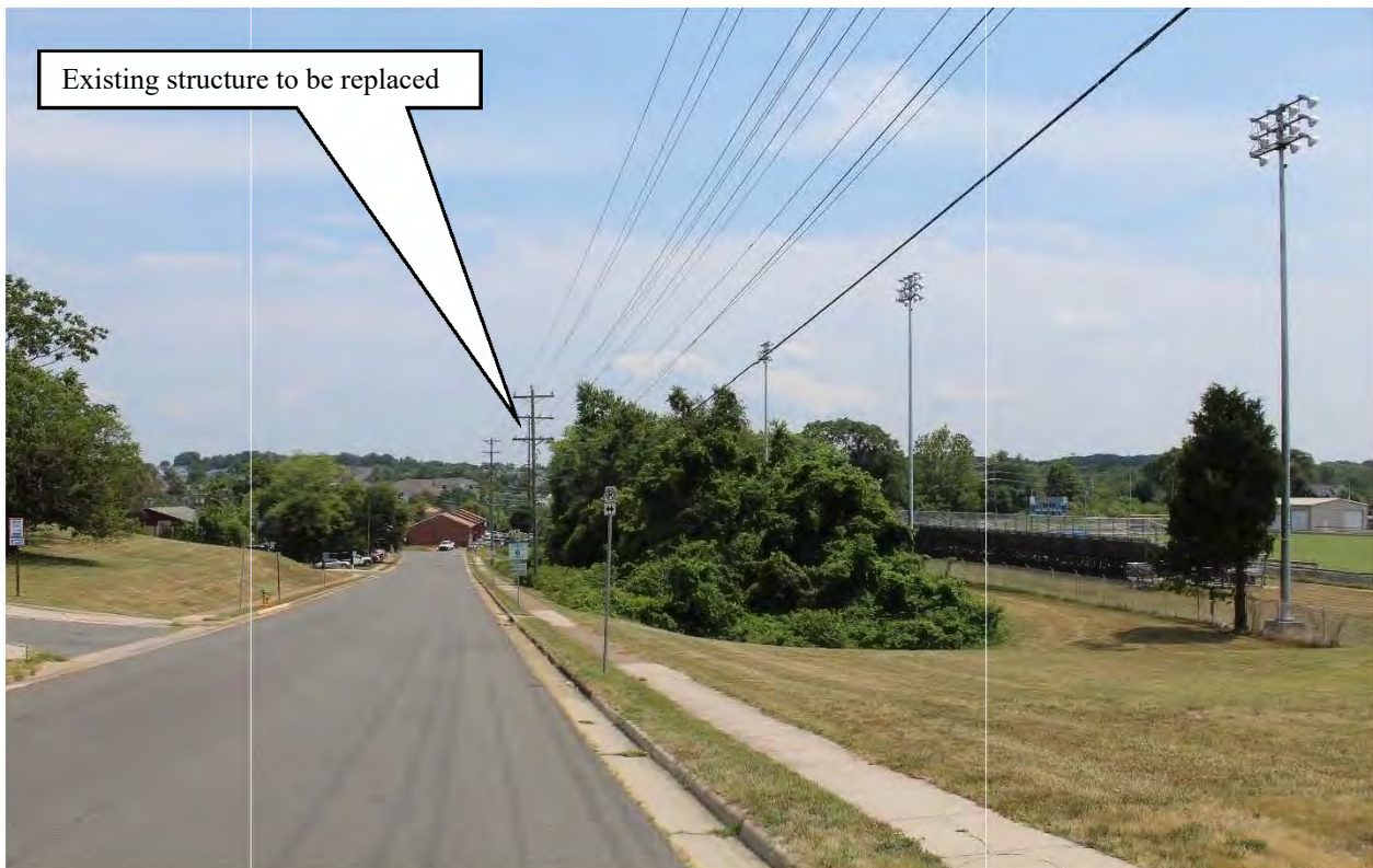
Figure 5-41: Photo location 4- View from Conner Drive at driveway to property (One project structure visible), facing southeast.
