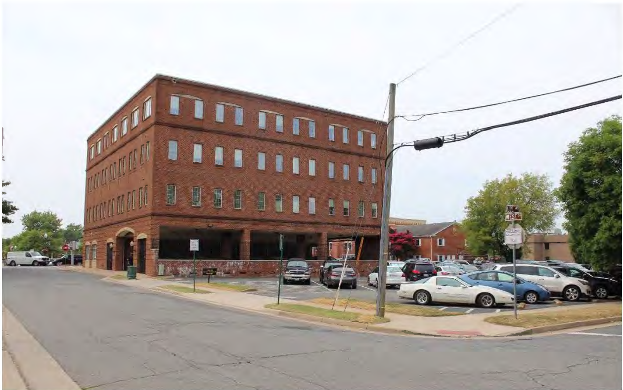
Figure 5-281: Photo location 1- Representative view of Pickeral House site (No project structures visible), facing southwest.
