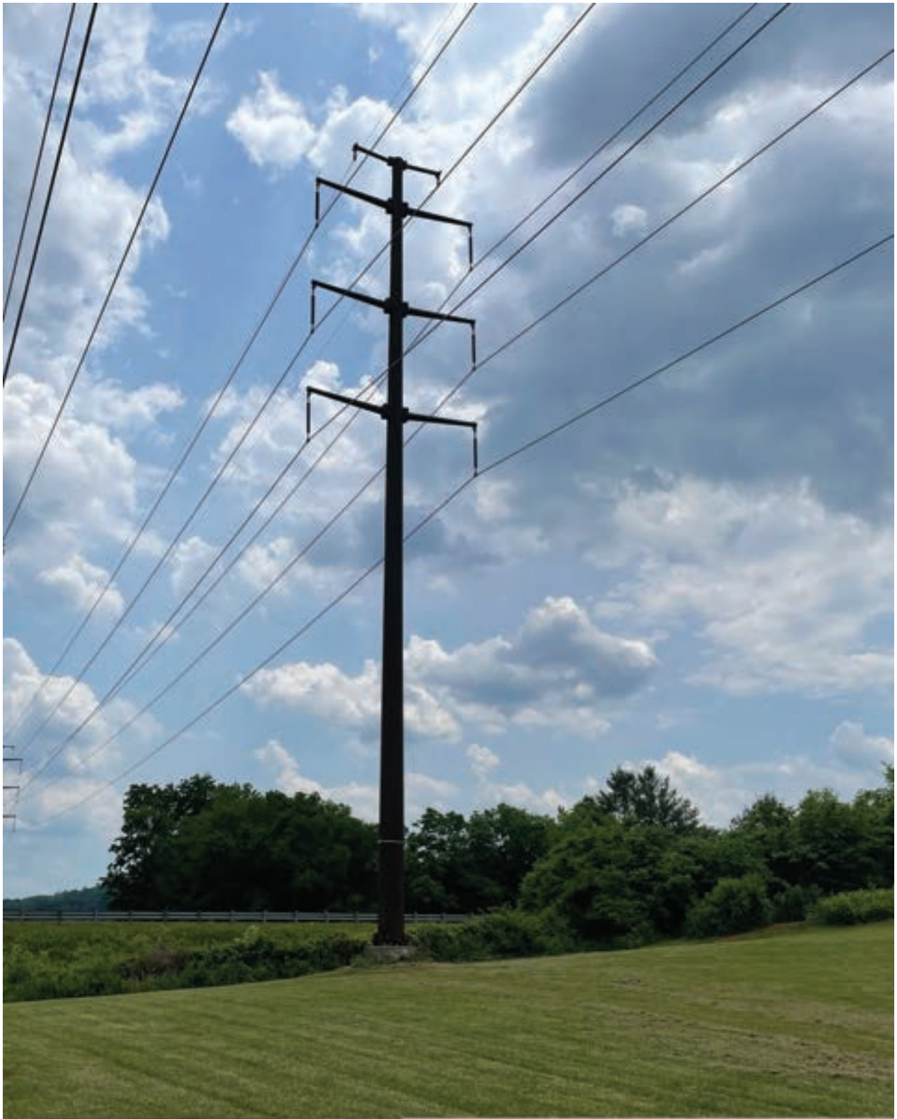
Existing Structure Type: 115 kV Double Circuit Steel Monopole (Tangent)
