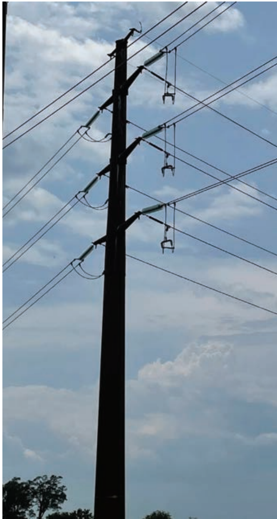
Existing Structure Type: 115 kV Double Circuit Steel Monopole (Modified Deadend )
