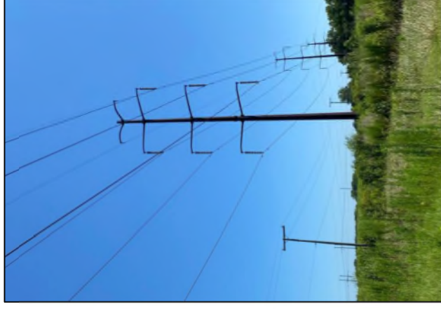
Examples of electric transmission double-circuit monopole structures. Not project specific.
