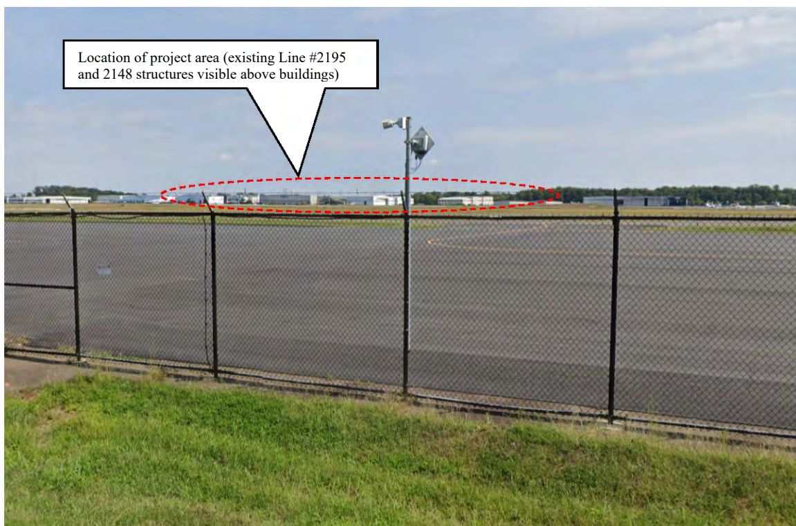
Figure 5-20: Photo location 1- View from Piper Lane at Manassas Regional Airport (Core Area) towards the project alignment (visible including structures on Line #2195 and 2148 within shared ROW), facing northeast.
