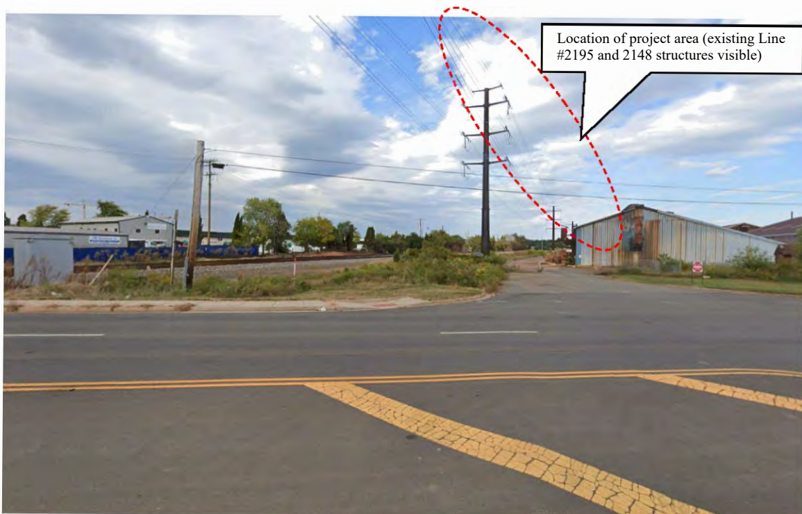
Figure 5-27: Photo location 8- View from Godwin Drive (Study Area) towards the project alignment (visible including several structures on Line #2195 and 2148 within shared ROW), facing north.
