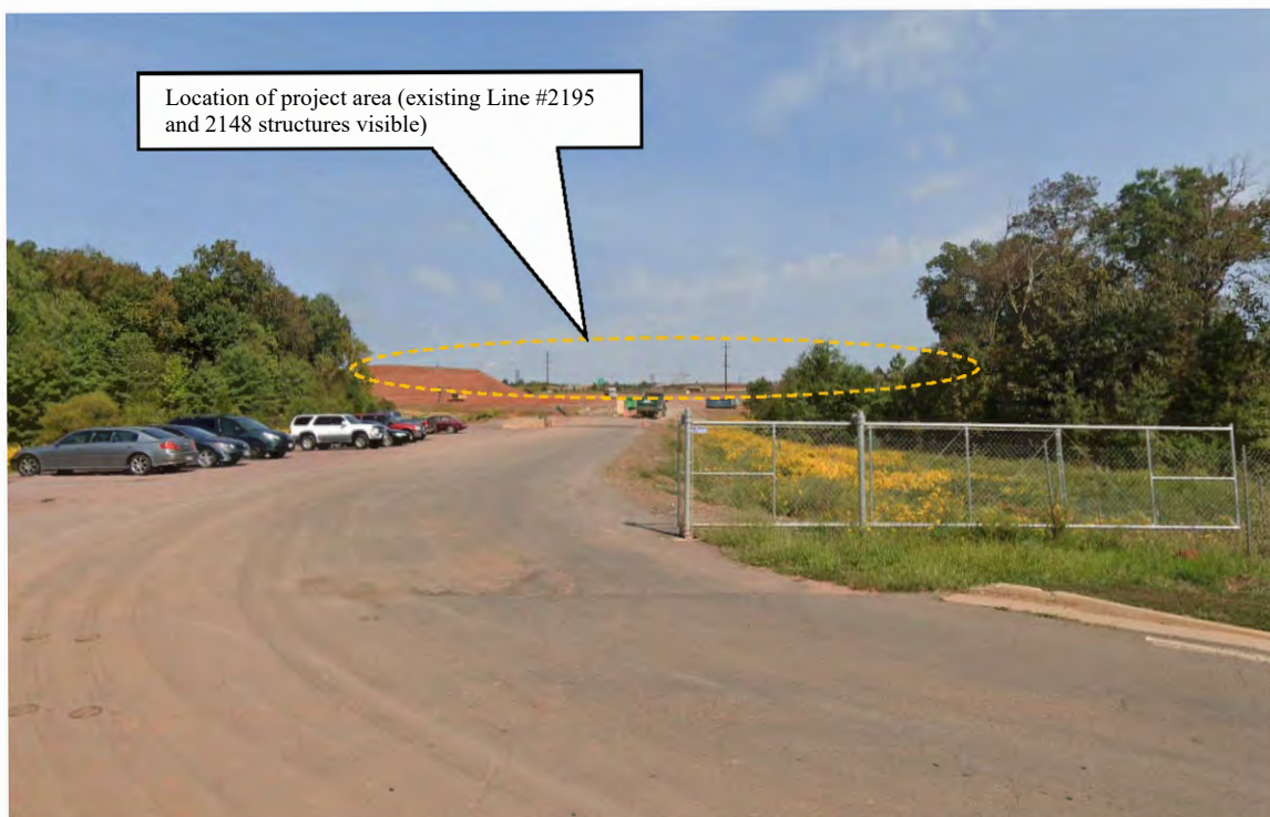
Figure 5-22: Photo location 3- View from Harry J Parrish Boulevard (Core Area) towards the project alignment (partially visible including several structures on Line #2195 and 2148 within shared ROW), facing northeast.
