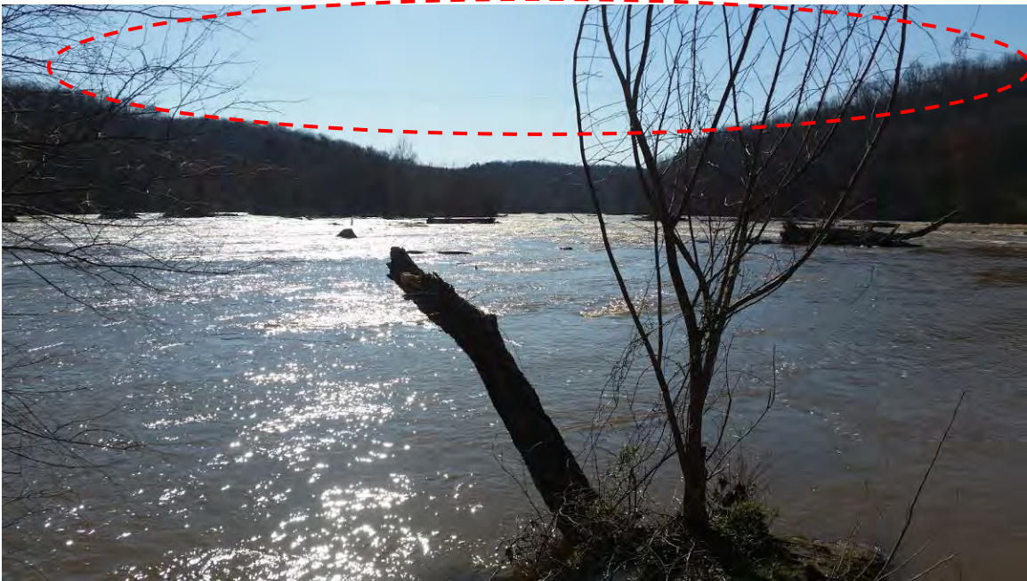
Photo 3: View from the confluence of the Rappahannock and Rapidan Rivers showing existing transmission line (red), facing east (Source: Waymarking.com)
