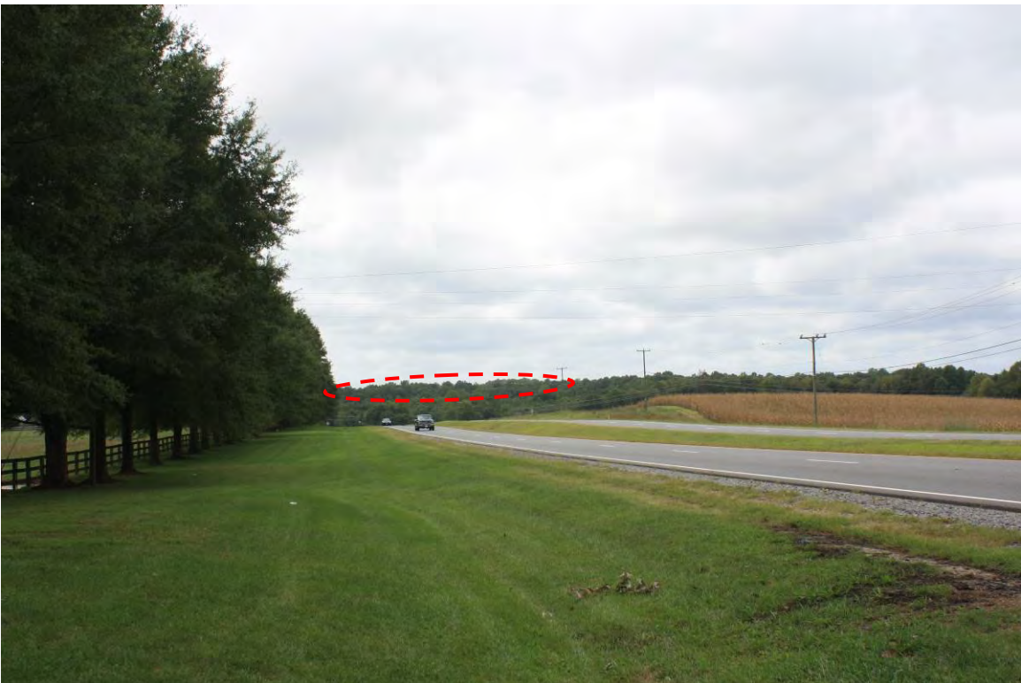
Photo 14: View from Courthouse Road (National Register Area) towards the existing transmission line (red), facing southeast
