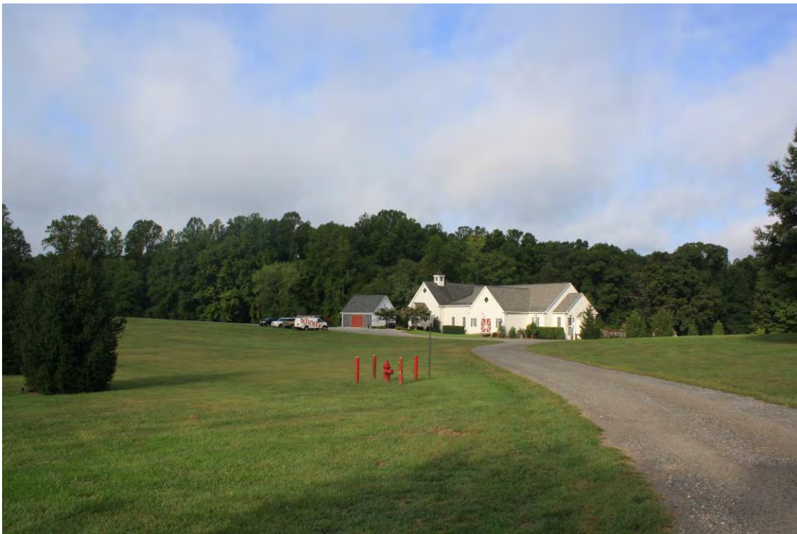
Photo 4: View of large modern barn, facing west
