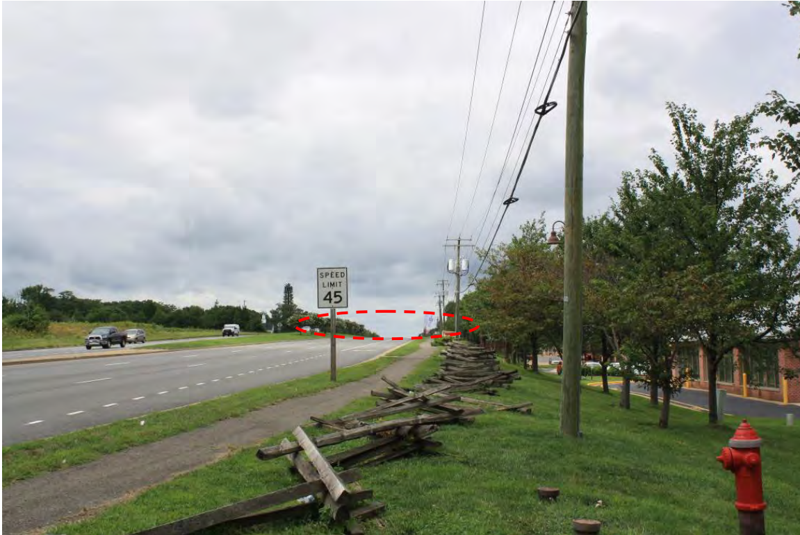
Photo 11: View from intersection of Plank Road and Harrison Road (study area) showing existing transmission line (red), facing west
