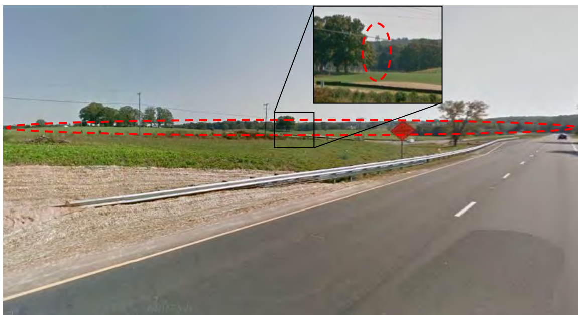
Photo 13: View from McLaws Drive showing the exiting transmission line (red) with detail of existing structure, facing northeast
