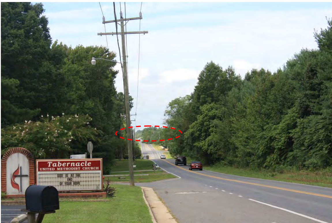
Photo 8: View from Old Plank Road (core area) showing existing transmission line (red), facing west
