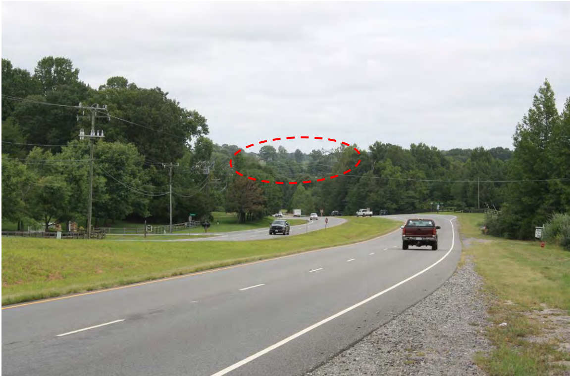
Photo 21: View from Courthouse Road showing one visible structure on exiting transmission line (red), facing northeast
