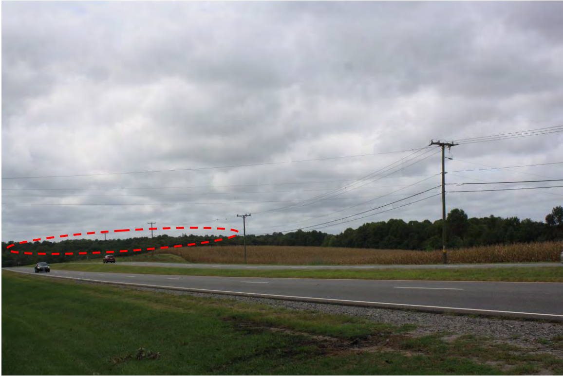
Photo 25: View from along Courthouse Road showing visible components of existing transmission line (red), facing west
