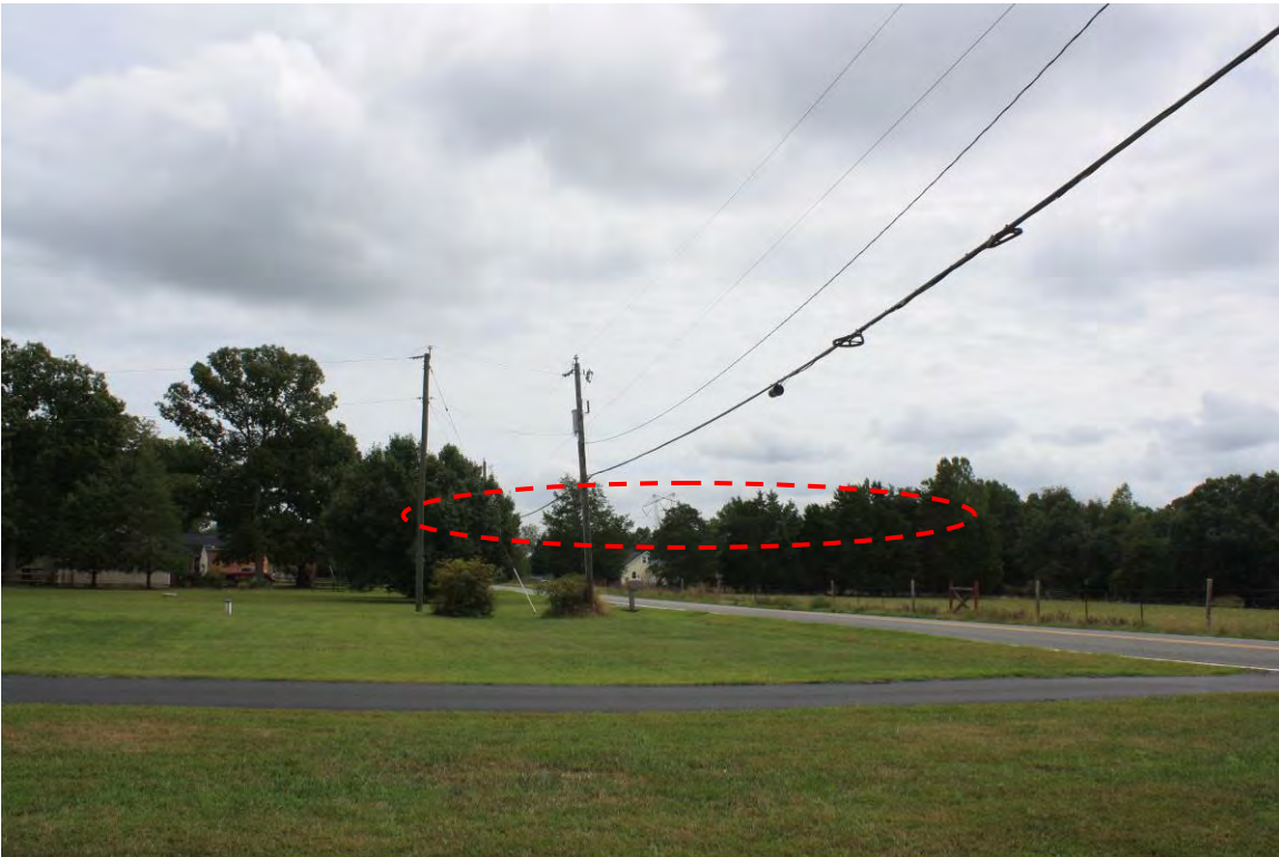
Photo 8: View from Massaponax Road (National Register area) towards the existing transmission (red), facing southeast
