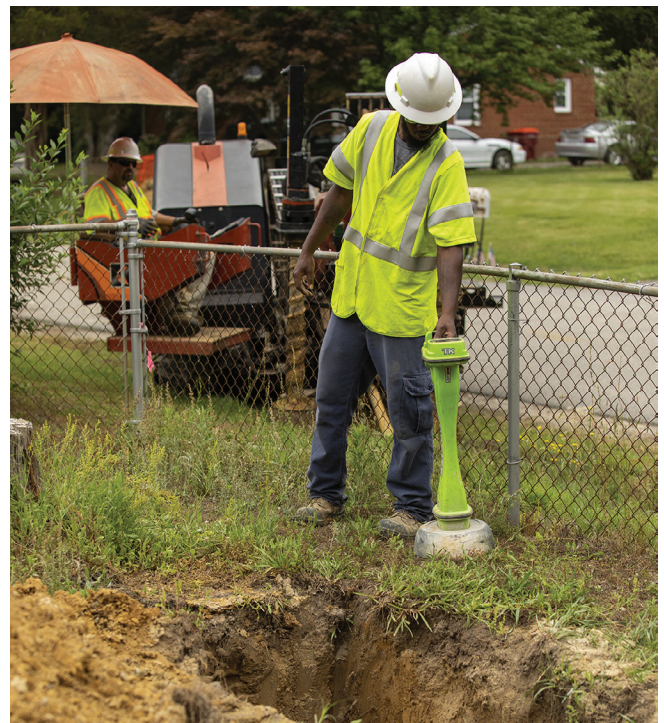
The contractor tracks the path of the drill under a fence.
