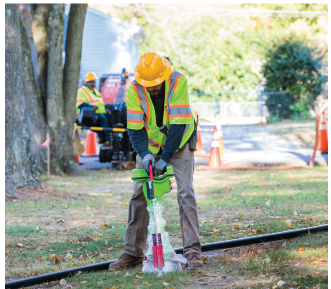
Another contractor tracks the path of the underground drill. The black conduit will be routed underground.
