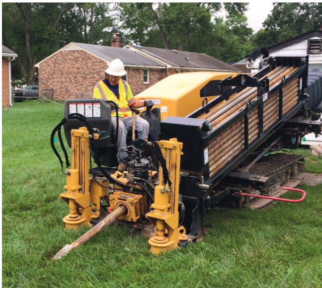
A Dominion Energy authorized contractor operates the underground directional boring equipment.
