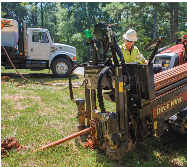
A tank of water is sometimes used to aid the drilling.
